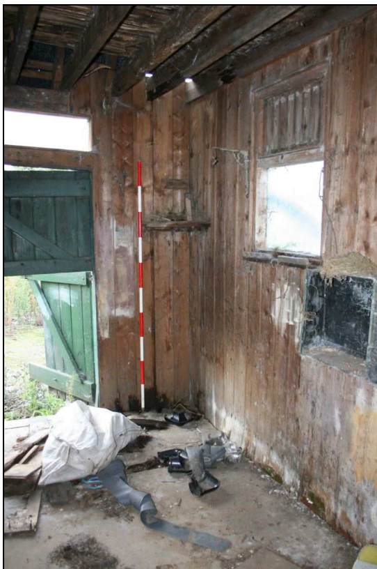
Plate 5: Room 1, view north-west
