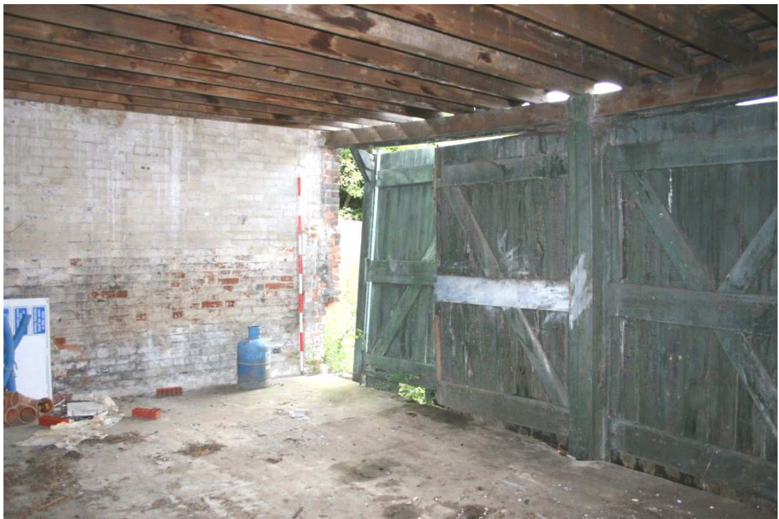
Plate 9: Room 3, view south-west
