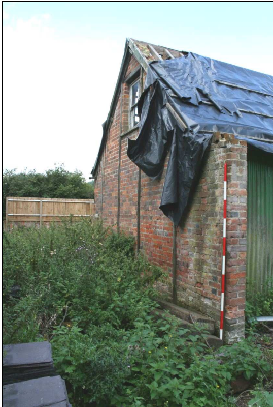
Plate 3: South elevation, from south-east
