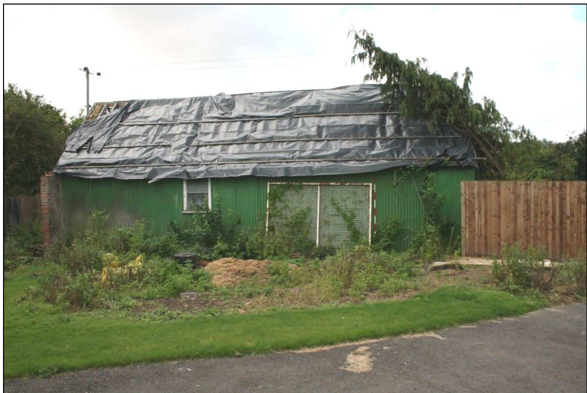
Plate 2: East elevation, from east
