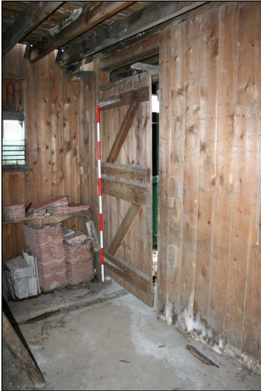
Plate 7: Room 2, view north-west
