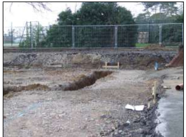
Plate 4: Sports centre trench, looking west
