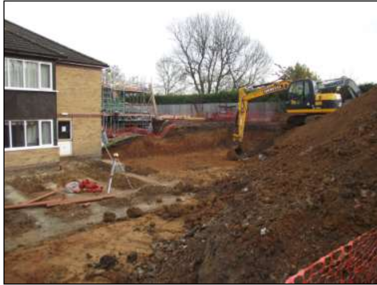
Plate 6: Extension B: north-western footings and ground reduction, looking E
