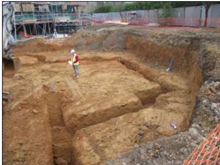
Plate 7: Extension B: ground reduction and south-eastern footings, looking NE
