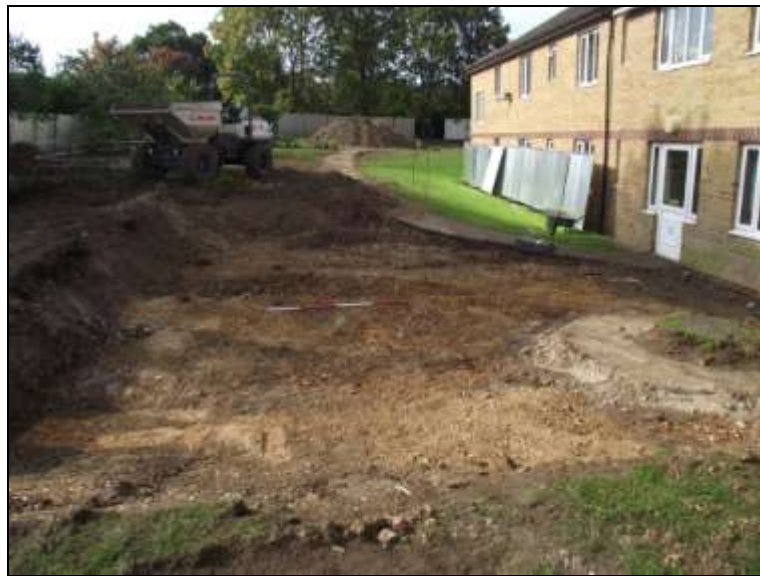
Plate 1: Extension A: ground reduction, looking SW ( scale 2m )
