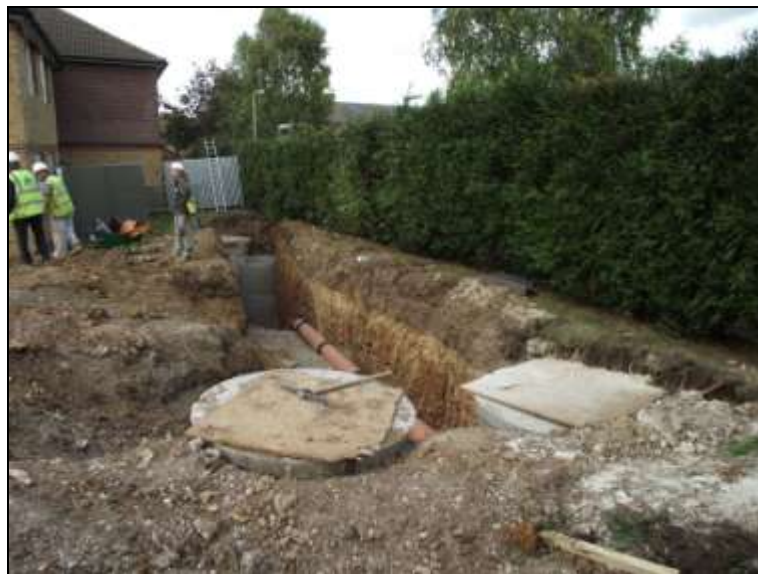
Plate 3: Drainage Trench, looking NW
