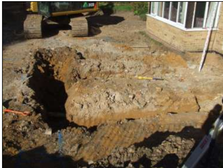
Plate 5: Extension B: footing trench, north-western end, looking NW
