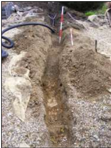
Plate 3: Cable trench, looking east
