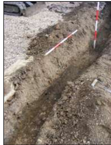
Plate 4: Cable trench, looking northeast
