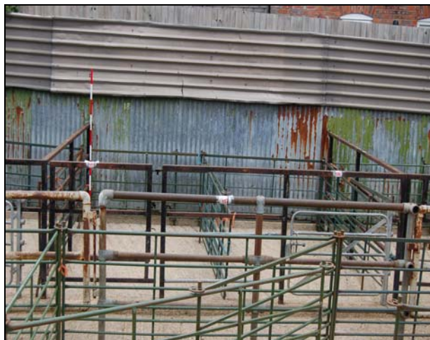
Plate 3: Area 1: Older pen along northern wall, looking north
