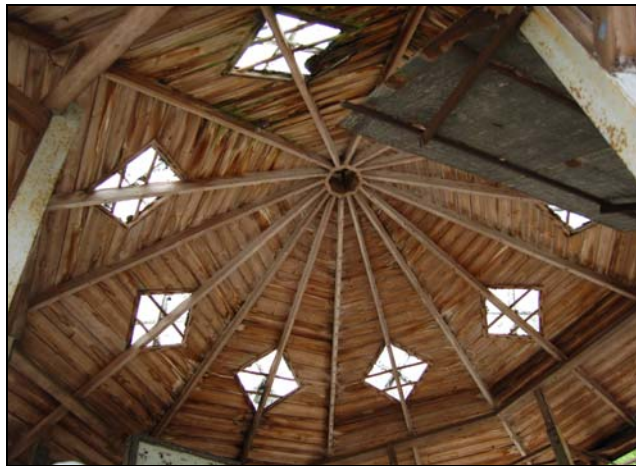
Plate 11: Area 1: Timber roof and cupola of auction ring
