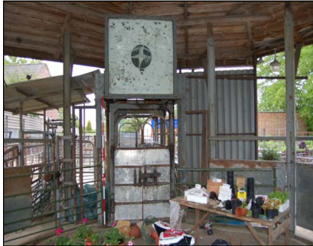
Plate 7: Area 1: Interior of former auction ring, showing cattle weighbridge, looking east
