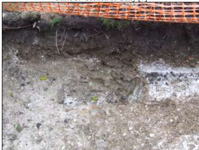
Plate 6: Section of Wall [9]
