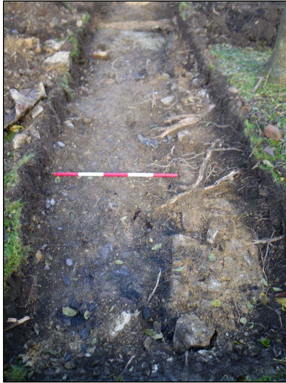
Plate 7: Wall [403] general shot looking north
