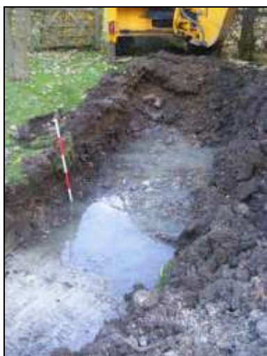
Plate 5: Soak away at Eastern end of Trench One, looking northeast
