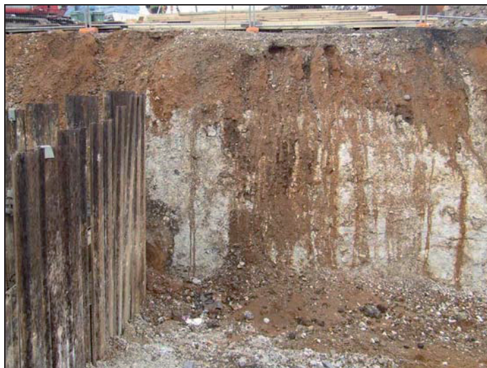
Plate 1: View of stratigraphy within cut for lower ground floor level
