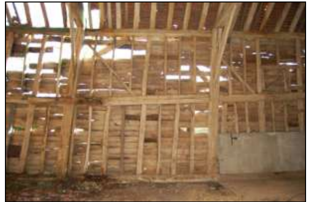
Plate 16: Main barn: Bay 6 south
