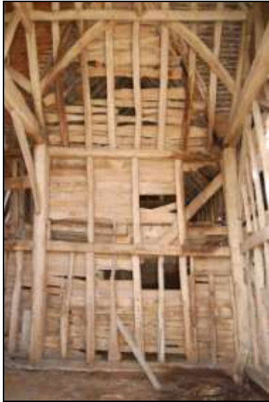
Plate 13: Main barn: Bay 7 north
