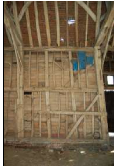
Plate 10: Main barn: Bay 4 north
