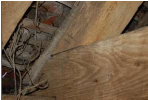
Plate 39: Carpenters assembly mark on roof truss
