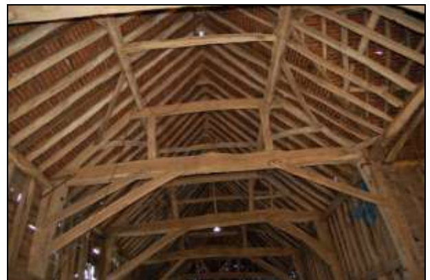
Plate 24: Main barn: Roof truss
