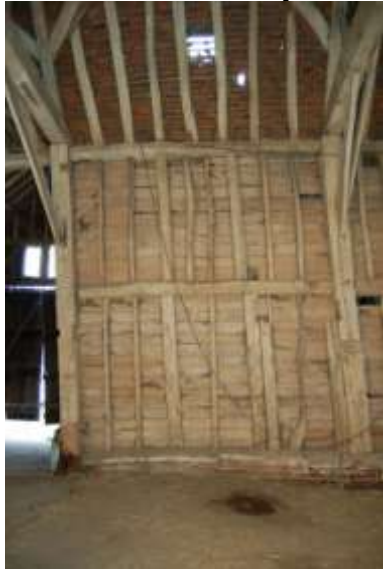
Plate 9: Main barn: Bay 3 north
