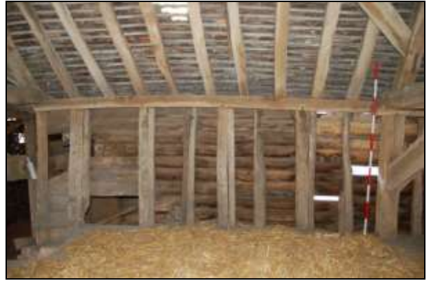
Plate 38: Upper floor southern end of west wall
