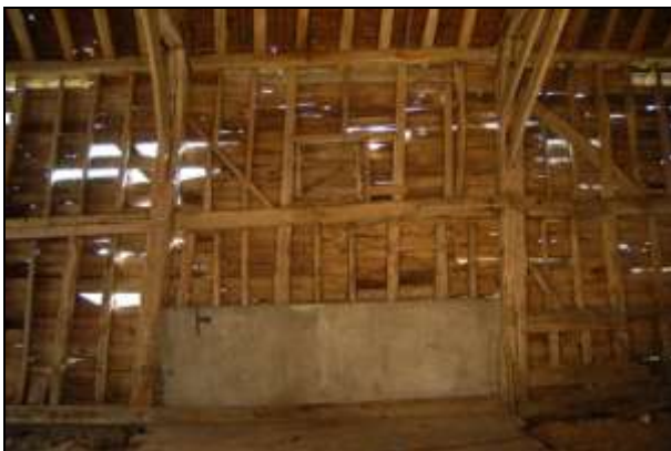
Plate 17: Main barn: Bay 5 south
