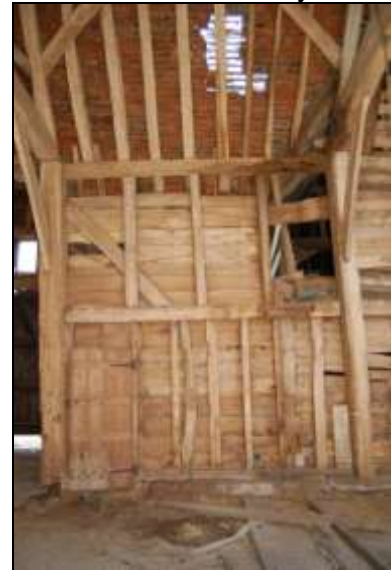
Plate 12: Main barn: Bay 6 north
