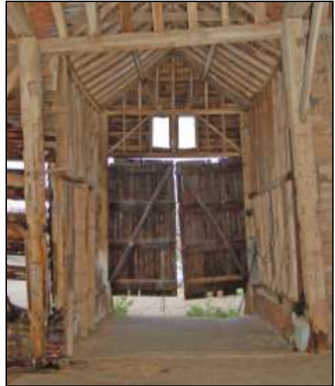
Plate 8: Main barn: Bay 2 north
