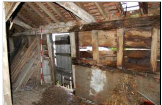
Plate 30: Western outshut north wall
