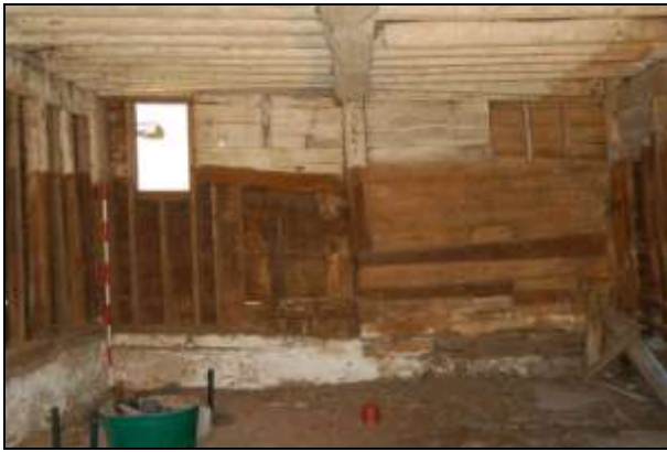
Plate 31: Eastern barn north wall
