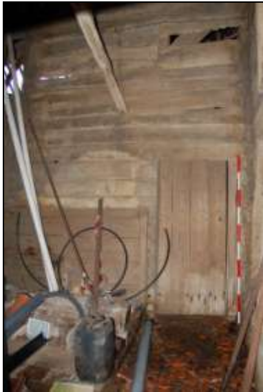
Plate 27: Eastern outshut south wall
