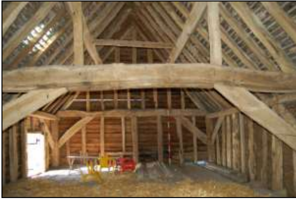
Plate 37: Upper floor north wall
