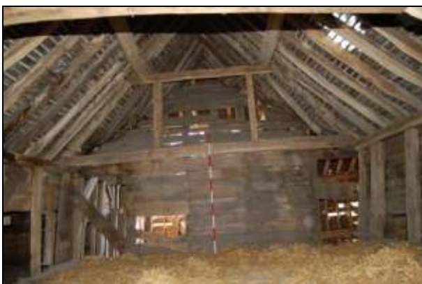
Plate 35: Upper floor south wall
