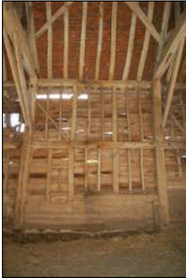
Plate 19: Main barn: Bay 3 south
