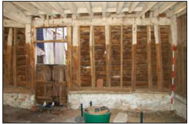
Plate 32: Eastern barn north end of west wall
