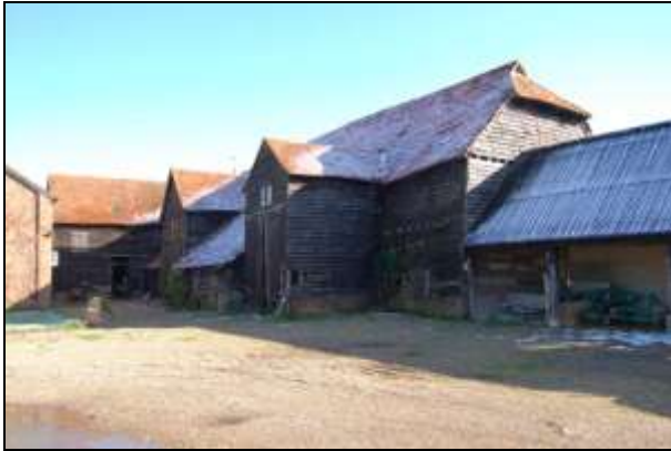
Plate 1: Barns form the northwest
