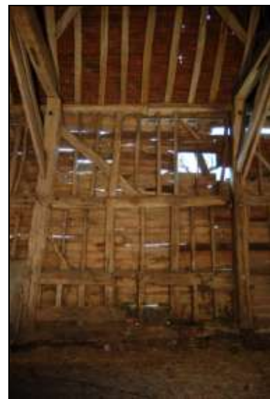
Plate 18: Main barn: Bay 4 south
