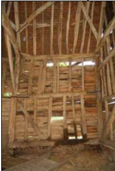
Plate 21: Main barn: Bay 1 south
