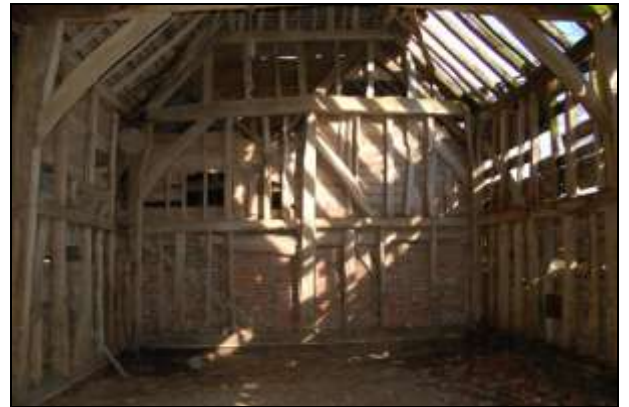
Plate 14: Main barn: East gable
