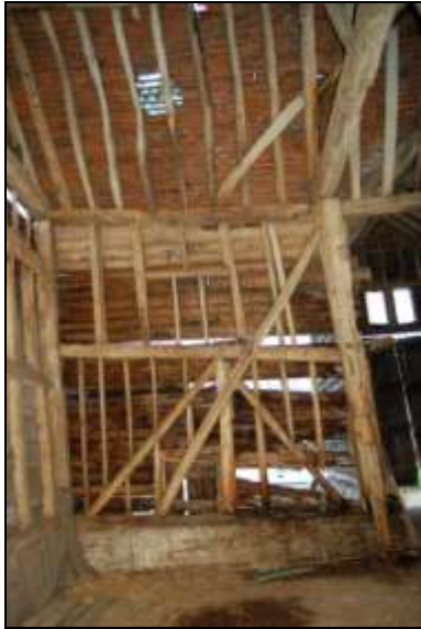
Plate 7: Main barn: Bay 1 north
