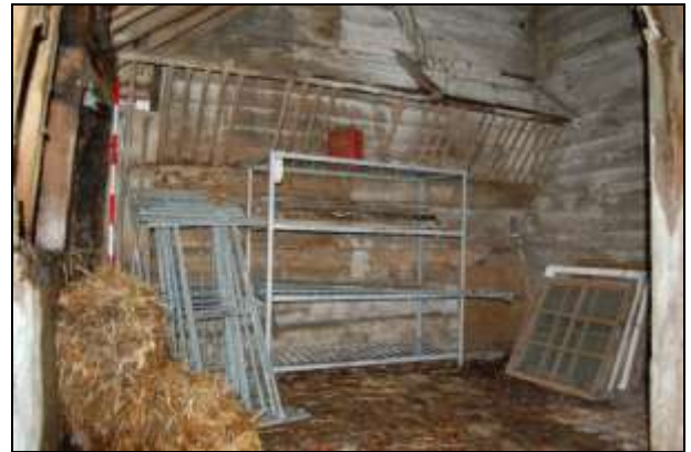
Plate 28: Western outshut east wall
