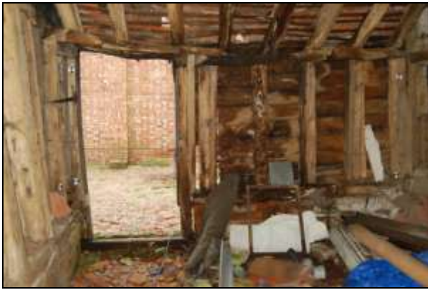
Plate 25: Eastern outshut north wall
