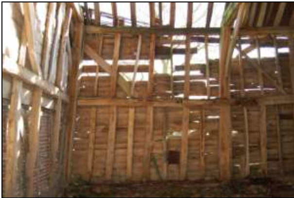
Plate 15: Main barn: Bay 7 south
