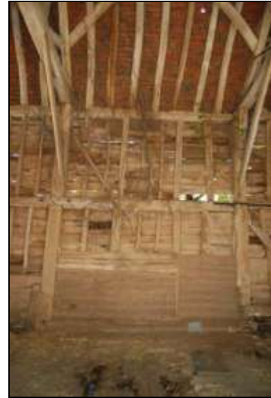
Plate 20: Main barn: Bay 2 south
