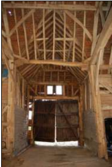
Plate 11: Main barn: Bay 5 north
