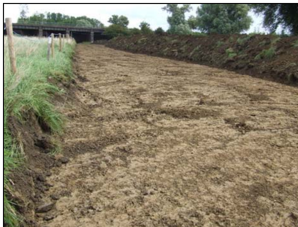
Plate 23: Overview of field west of bridges
