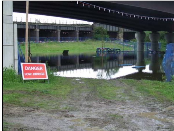
Plate 1: View of flooding constraints below A6 bridge
