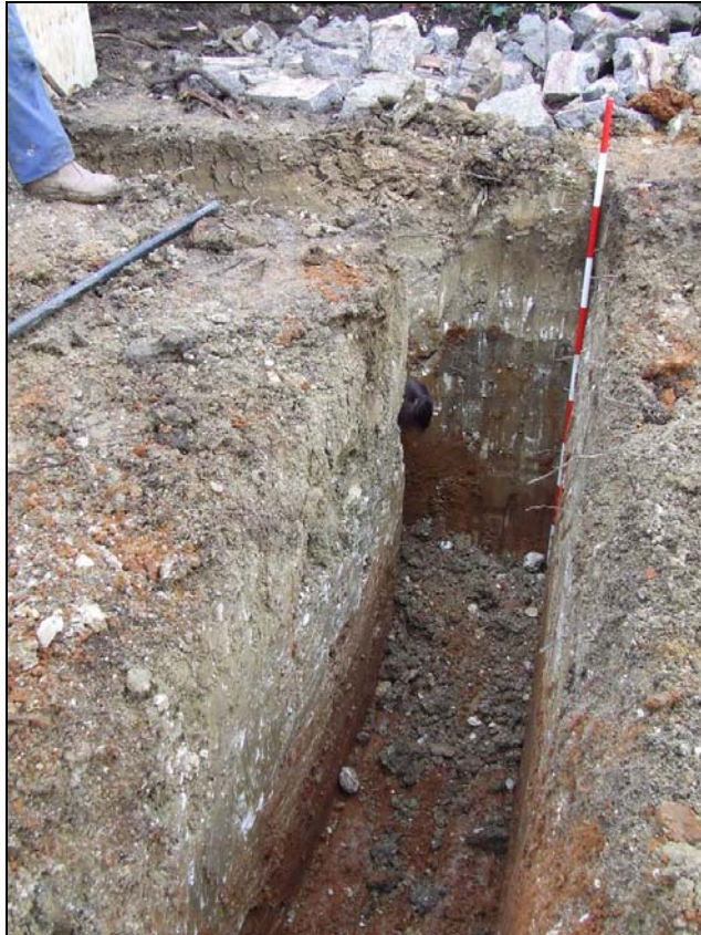
Plate 1: Footing trench, looking north, 2m scale
