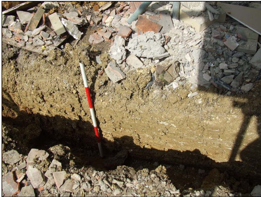
Plate 3: Conservatory footing trench, looking north, 1m scale
