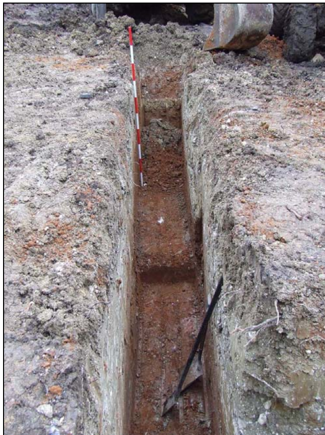
Plate 2: Footing trench, looking west, 2m scale
