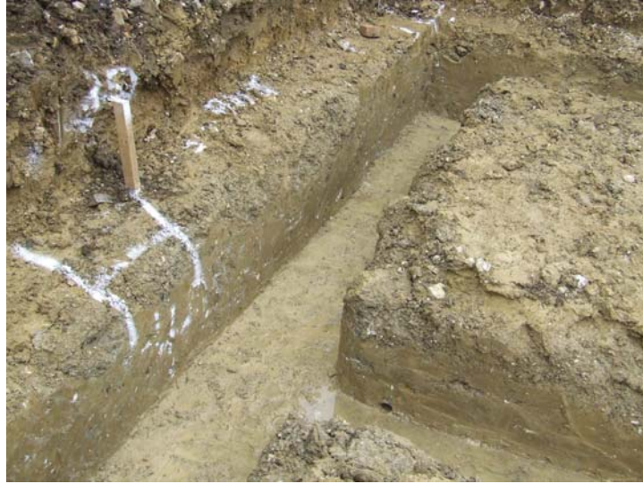
Plate 1: Typical section of footings
