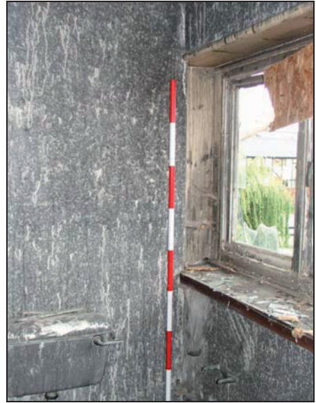
Plate 62: F7, looking north-west
