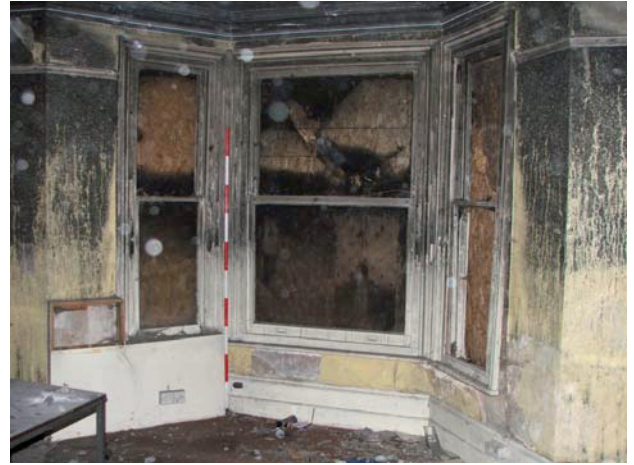
Plate 50: G5, bay window looking south-east
