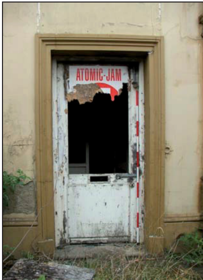
Plate 6: South elevation, detail of front door (G1)
