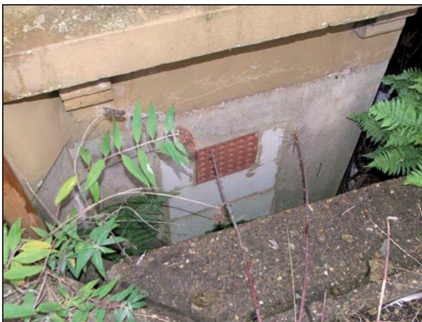
Plate 8: South elevation, detail of lower section of bay window (C7)
