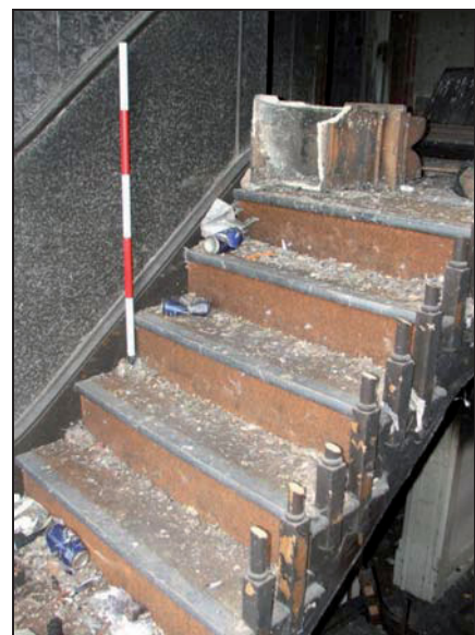
Plate 36: F1, stairs above half landing
