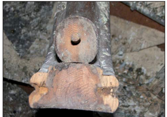
Plate 38: G1, section through stair handrail
