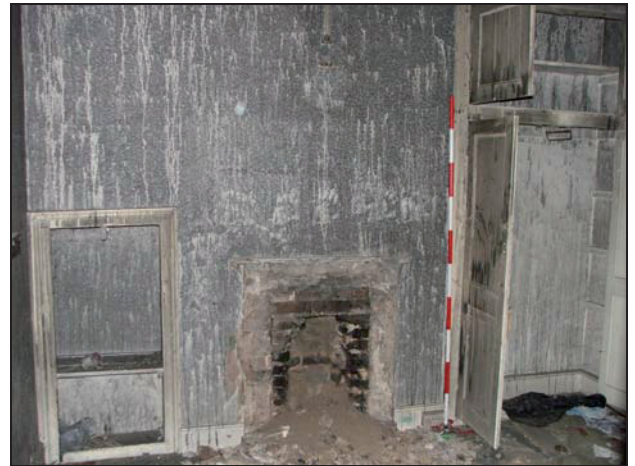
Plate 64: F9, looking east
