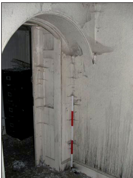
Plate 59: F4, detail of arch and door casing to F3
