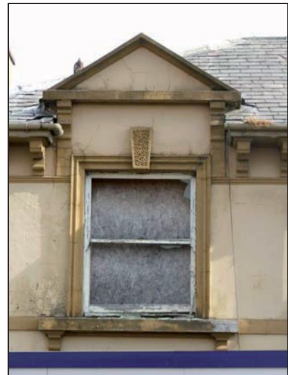
Plate 5: South elevation, detail of first-floor window (F4)
