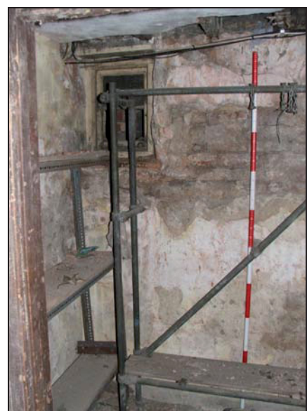
Plate 24: C6, looking south-east
