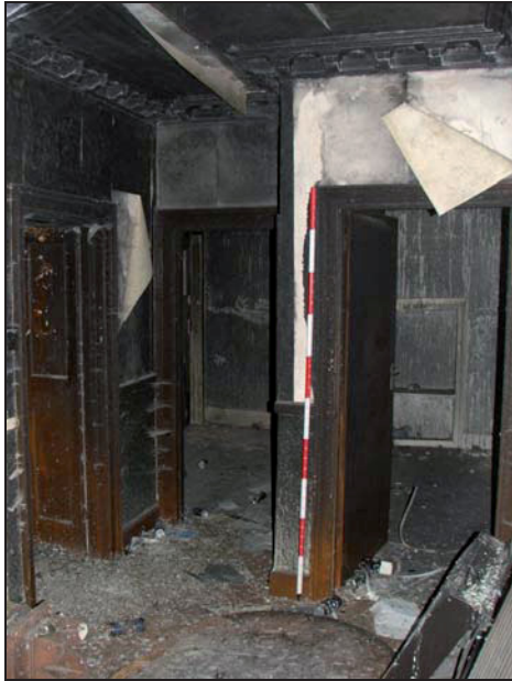
Plate 55: F1, looking east
