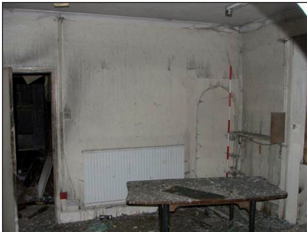
Plate 57: F4, looking east
