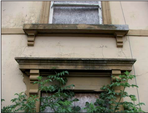
Plate 4: South elevation, detailing above and below windows (G2 & F4)
