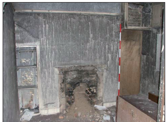
Plate 60: F5, looking west
