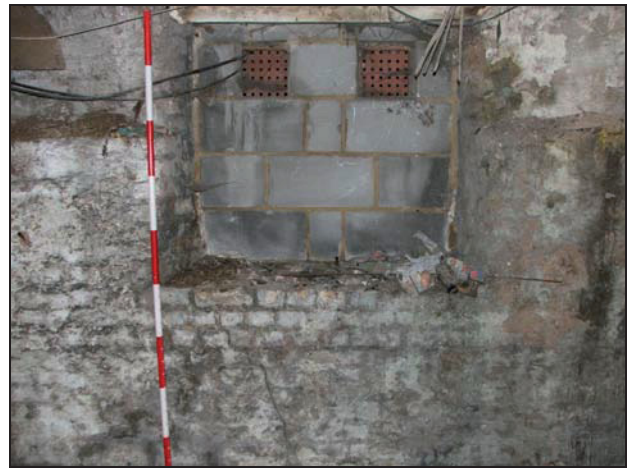
Plate 20: C4, looking south (blocked window)
