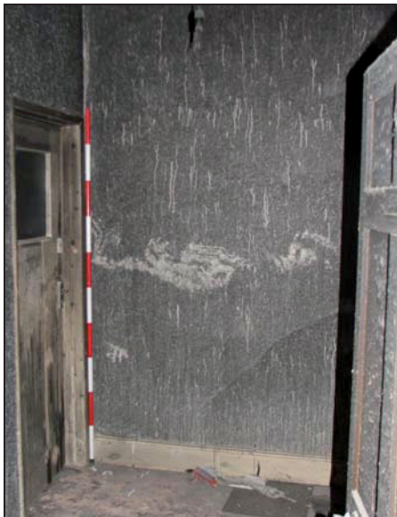
Plate 63: F8, looking east
