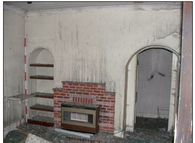
Plate 58: F4, looking west
