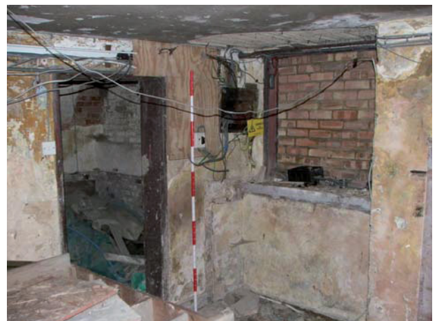
Plate 28: C7, looking north-east (doorway & blocked window)
