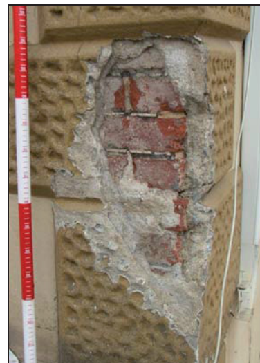
Plate 9: North elevation, tuck pointing under applied quoin on SE corner
