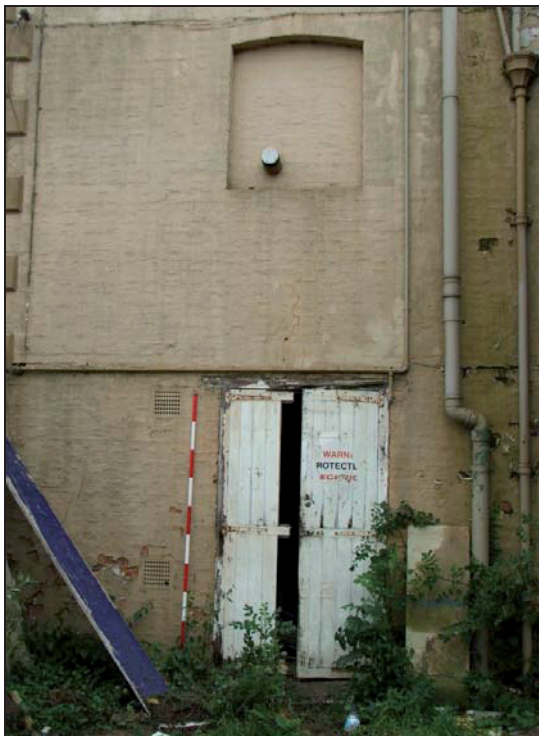
Plate 11: North elevation, detail of east part
