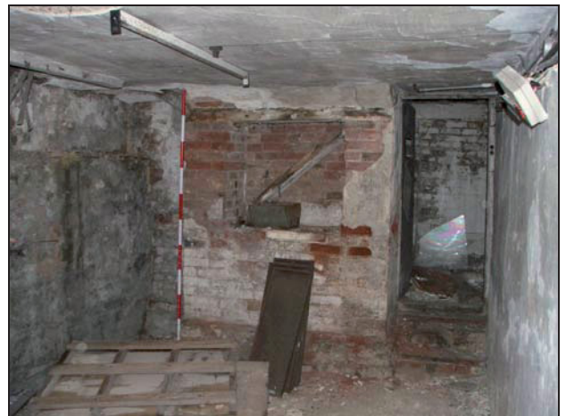
Plate 22: C4, looking west (base of chimney stack)
