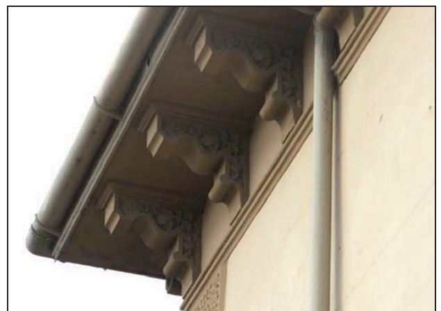
Plate 3: Detail of eaves brackets
