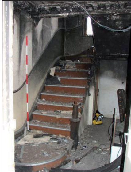
Plate 31: G1, looking north (stairs)
