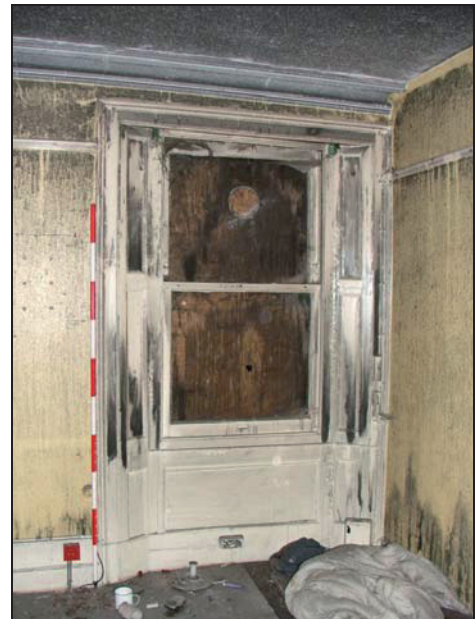
Plate 52: G6, window looking south-east
