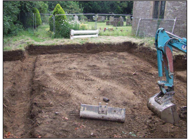
Plate 2: Overview of site after digging foundations
