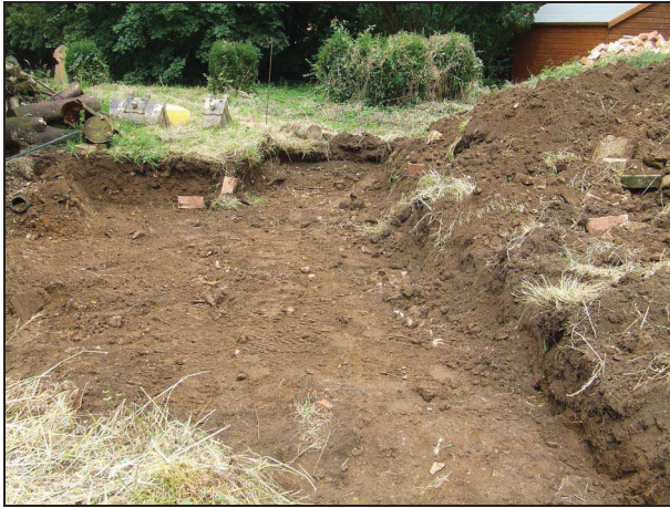
Plate 1: Overview of site during ground reduction
