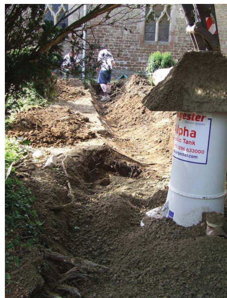
Plate 12: Excavating drain to new septic tank
