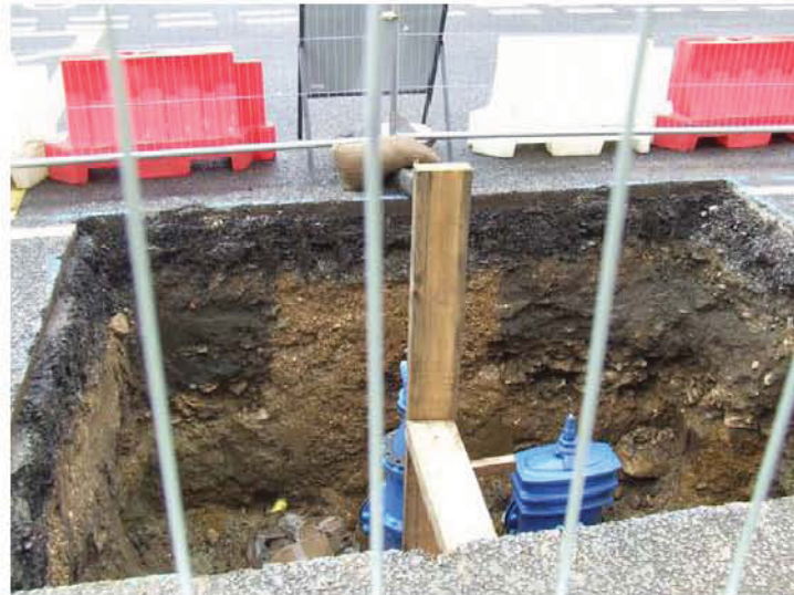
Plate 4: 19 th century deposit/feature in Area 4.
