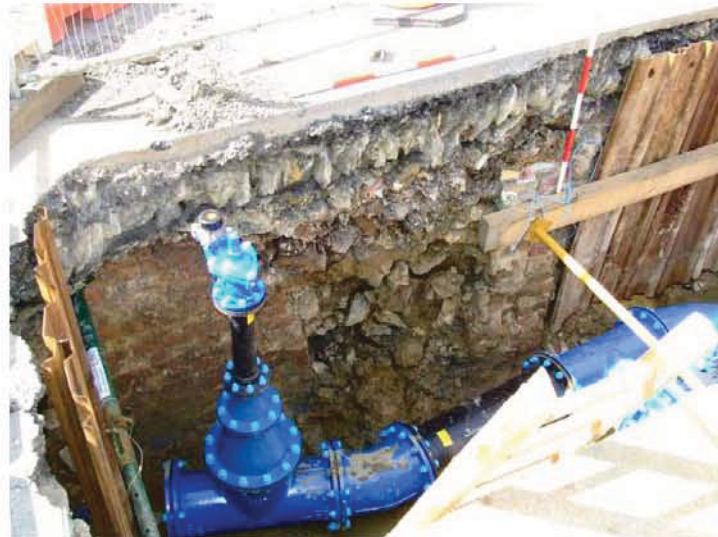
Plate 5: 20 th century brick built inspection chamber in Area 5.
