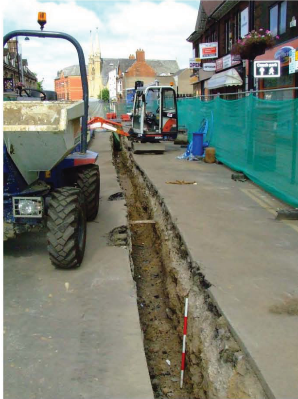
Plate 7: Trench east of Lincoln Road revealing earlier surfaces.
