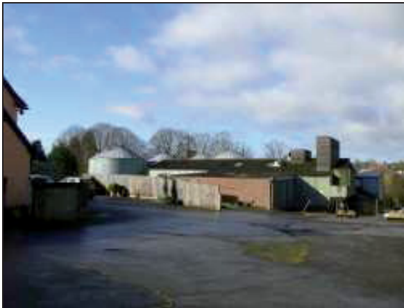
Plate 9: Buildings 6-7 and silos looking south west towards St Marys
