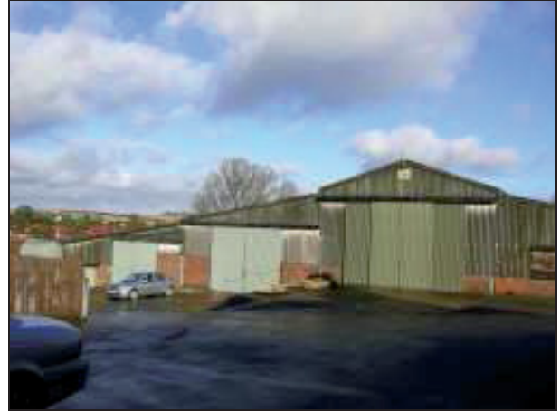
Plate 8: Southern end of modern buildings B4 and B5
