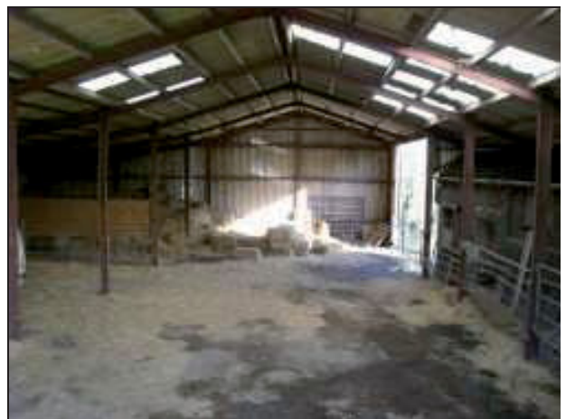
Plate 6: Internal view of B2
