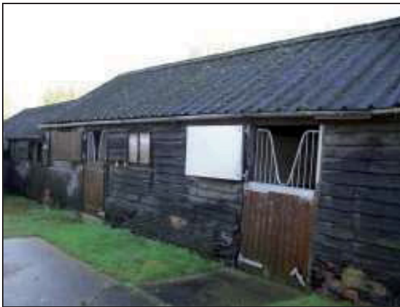
Plate 3: Timber stables (B1)
