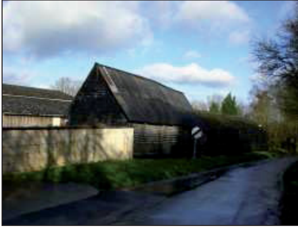
Plate 1: Timber building (B1) looking north from lane
