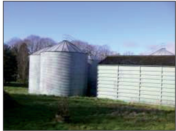
Plate 10: View south west across corn silos (B8)
