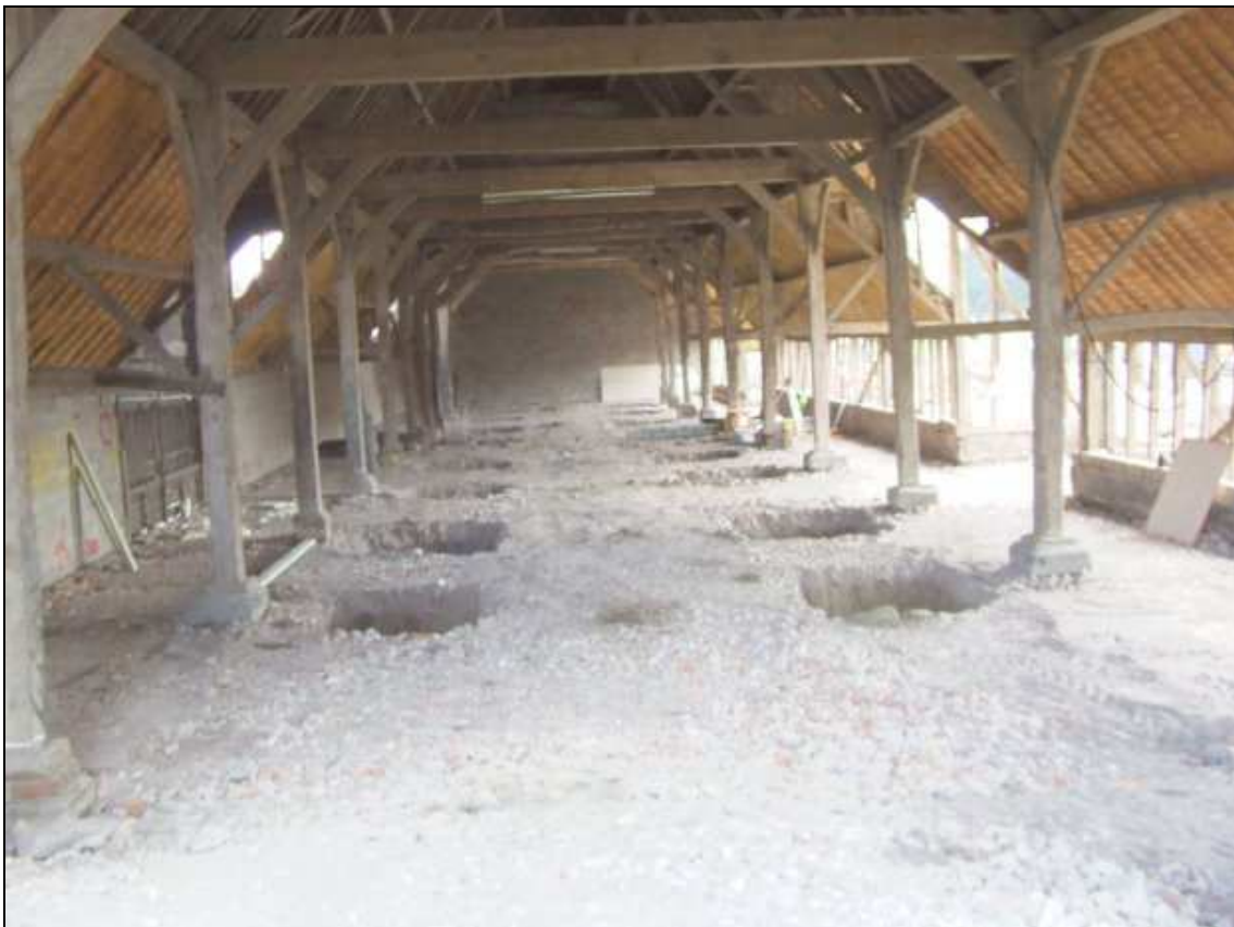
Plate 1: Excavated pits for the mezzanine floor supports in the northeastern barn
