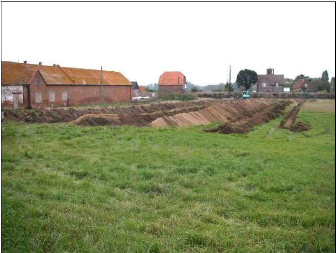
Plate 5: Location of the geo-thermal pipe trenches
