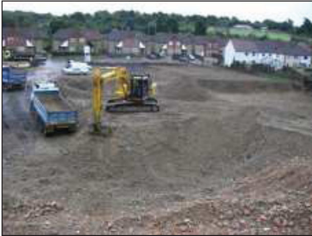
Plate 1: General view of site, illustrating constraints on the evaluation
