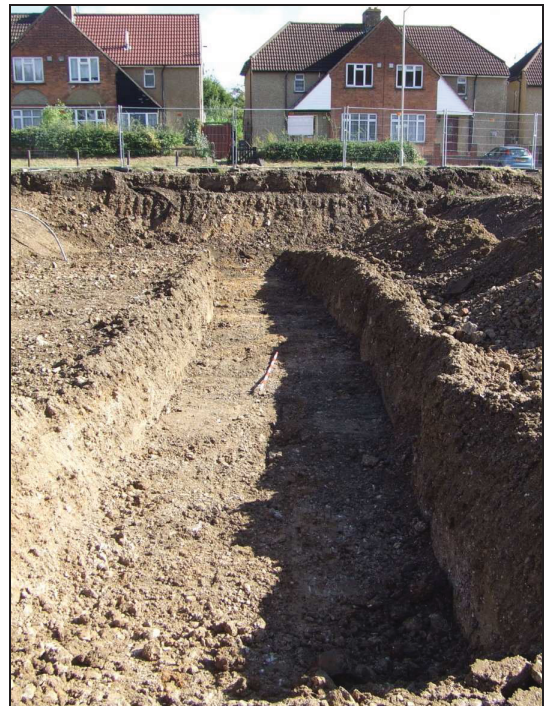
Plate 4: Trench 5 from west, scale 2m
