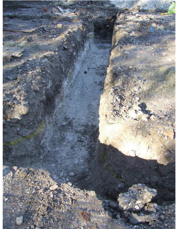
Plate 2: Typical footing trench section
