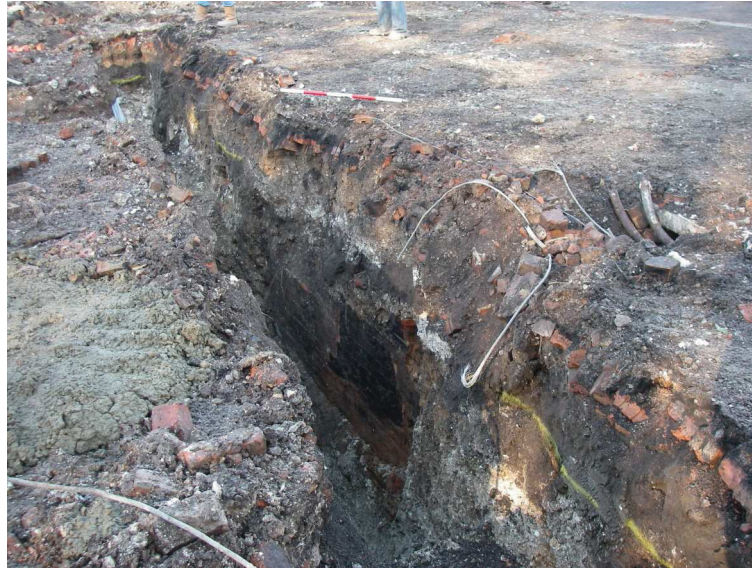
Plate 6: Cellars in eastern footing trench
