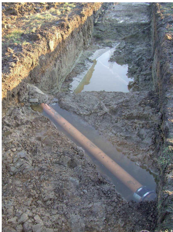
Plate 4: Constraints in Trench 2 (repaired land drain)
