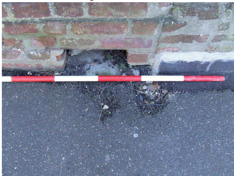
Plate 17: Detail of drain in base of wall adjacent to 17 High Street
