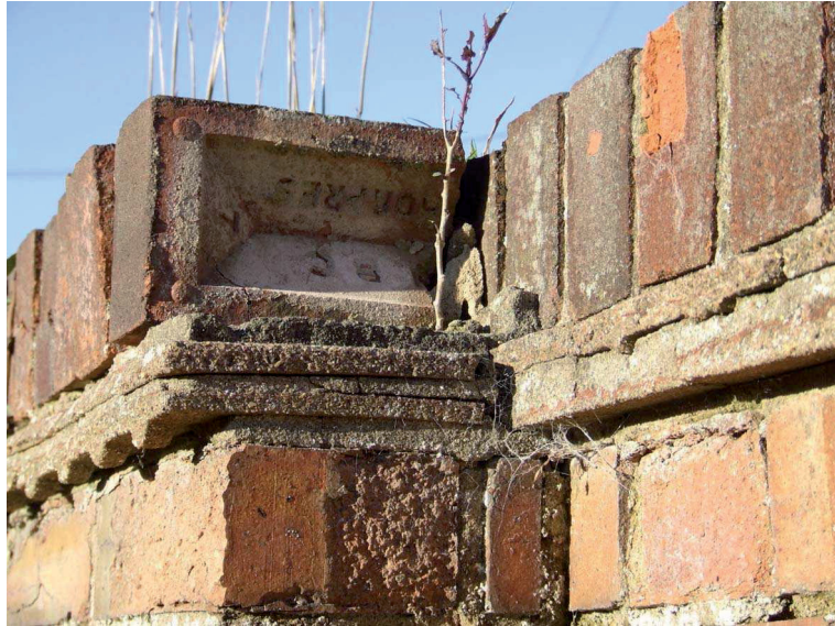
Plate 15: Detail of capping to modern section of wall
