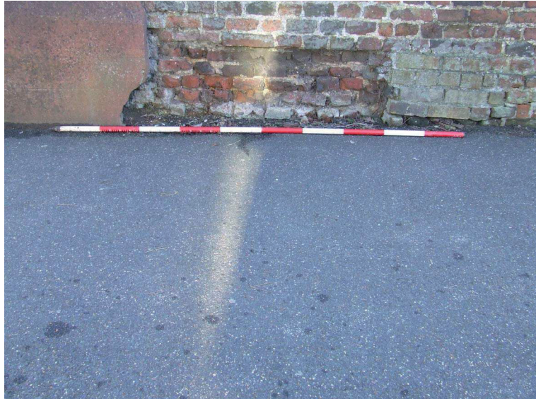
Plate 16: Detail of frost damage and repairs, showing older part of wall continuing behind concrete render.
