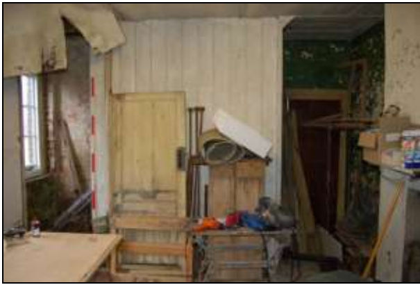
Plate 7: Room G1: north wall
