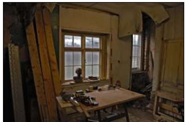
Plate 6: Room G1: west wall
