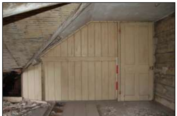
Plate 18: Room F2: north wall
