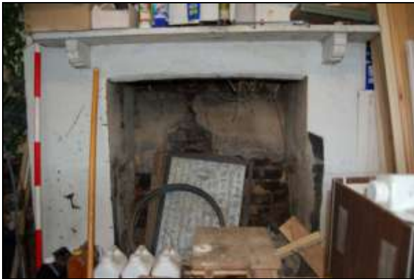
Plate 9: Room G1: fireplace detail
