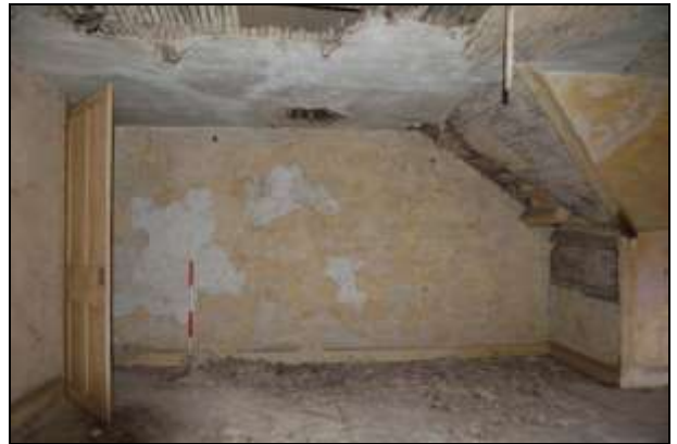
Plate 16: Room F1: north wall
