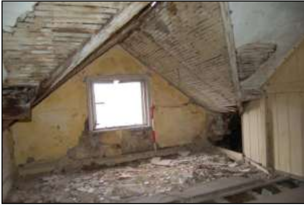
Plate 19: Room F2: west wall
