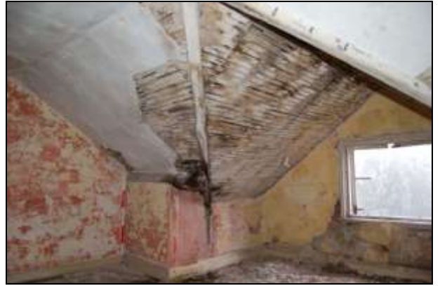
Plate 20: Room F2: southwest corner
