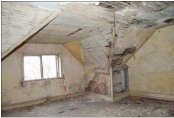
Plate 13: Room F1: southeast corner
