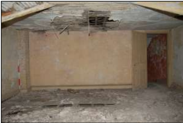
Plate 15: Room F1: west wall
