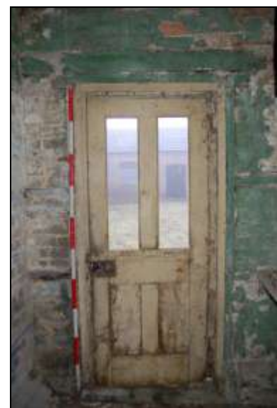
Plate 12: Room G2: looking west
