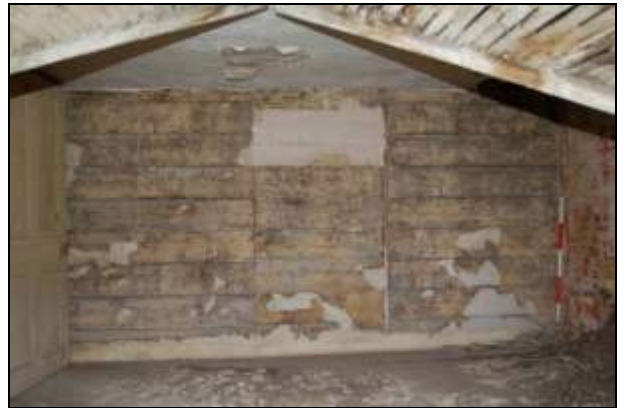
Plate 22: Room F2: east wall
