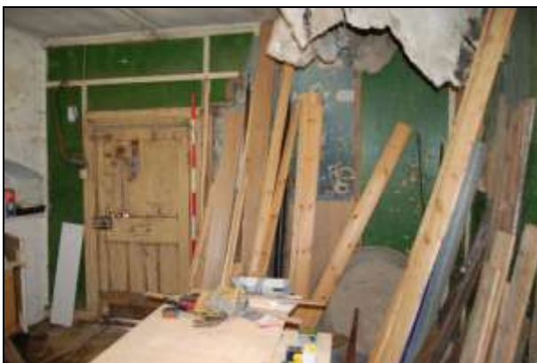
Plate 5: Room G1: south wall
