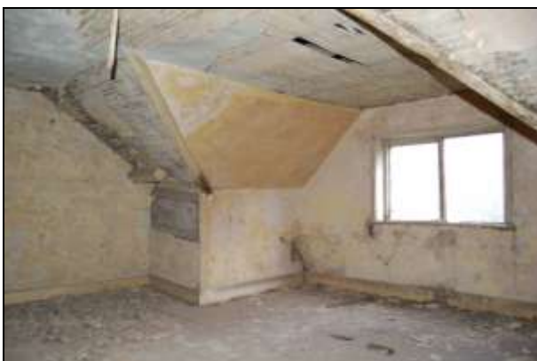
Plate 17: Room F1: northeast corner
