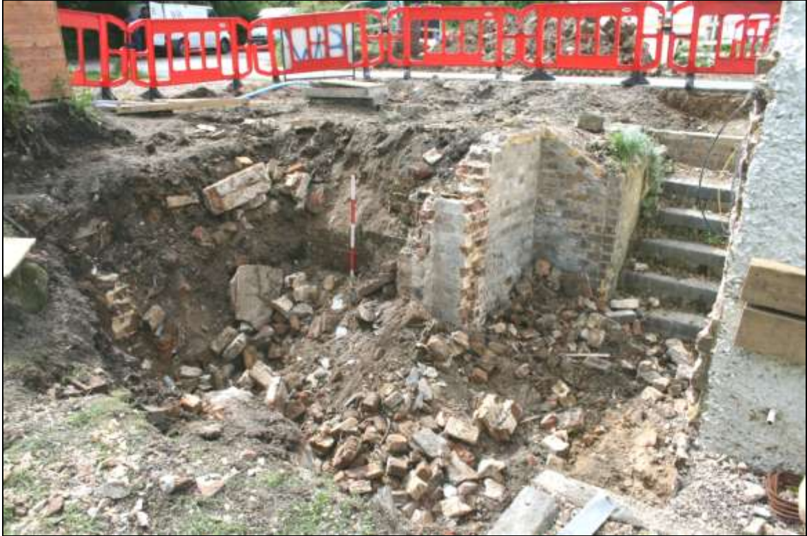
Plate 2: Site during excavation: scale on north-west side of additional room
