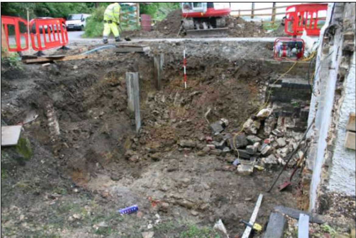
Plate 3: Site following removal of brick cellar structures
