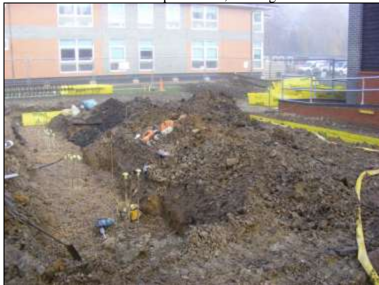
Plate 3: General shot, looking north
