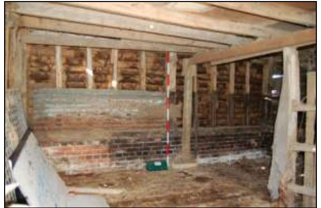
Plate 4: Bay 1: west wall
