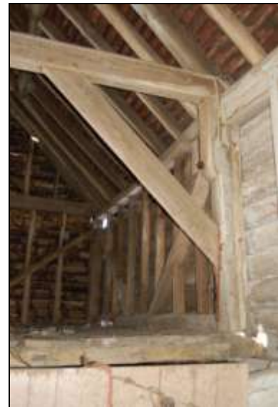
Plate 10: Bay 1: north wall above mezzanine floor
