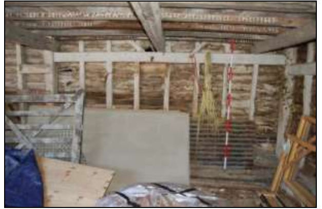
Plate 14: Bay 3: north wall
