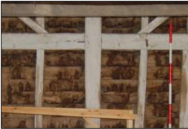
Plate 19: East wall showing chamfer detail
