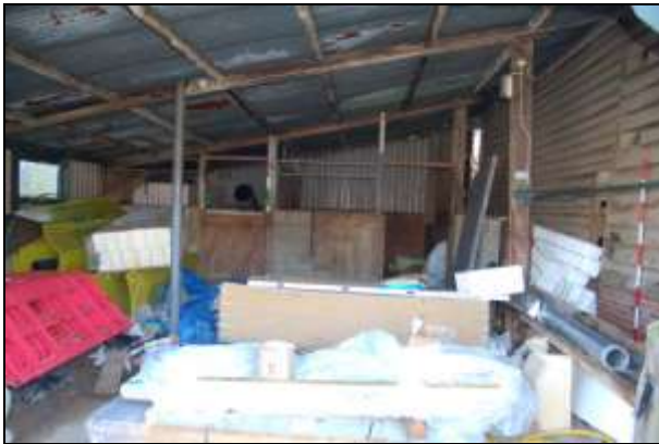
Plate 21: Interior of modern addition looking east
