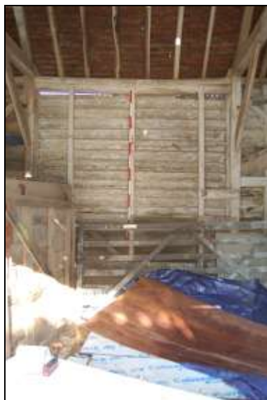
Plate 11: Bay 2: north wall
