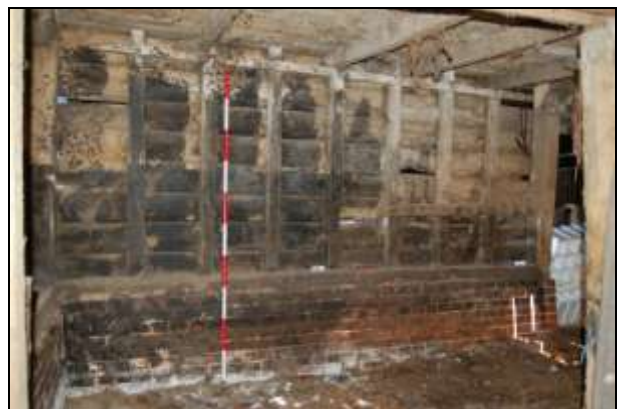
Plate 6: Bay 1: north wall
