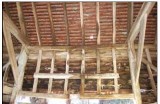
Plate 12: Bay 2: south wall showing jowlpost detail
