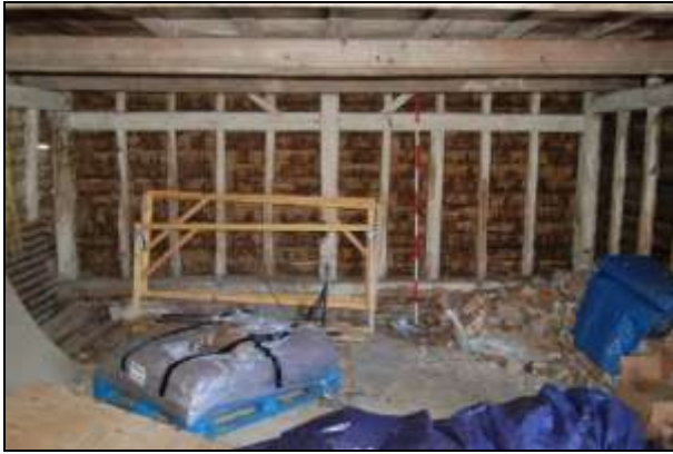
Plate 13: Bay 3: east wall
