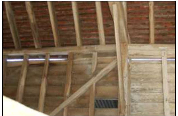
Plate 20: Counterbladed scarf joint in north wall
