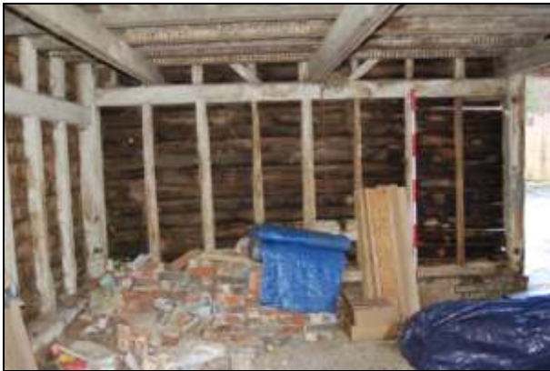
Plate 15: Bay 3: south wall
