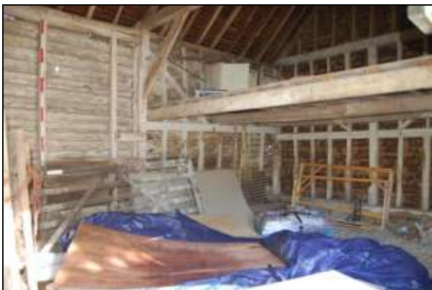
Plate 17: Bay 3: northeast corner
