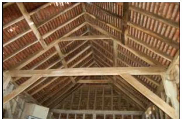
Plate 18: Eastern truss
