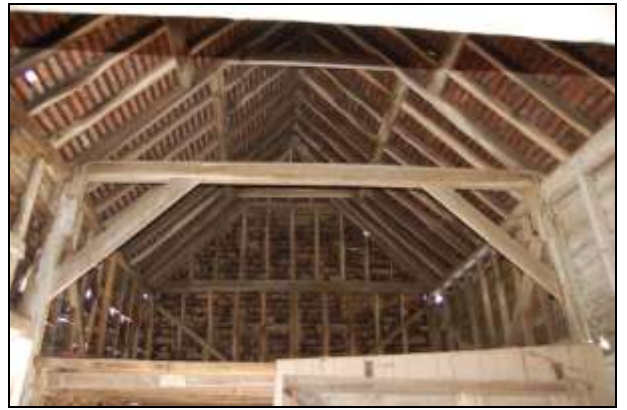
Plate 8: Bay 1: west wall above mezzanine floor
