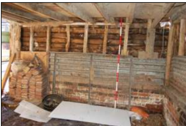
Plate 5: Bay 1: south wall
