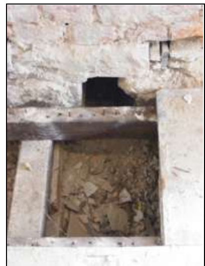
Plate 6: Internal exit point of drain, running out of the kitchen
