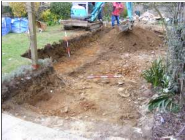
Plate 1: Development area, looking southwest 2x1m scale
