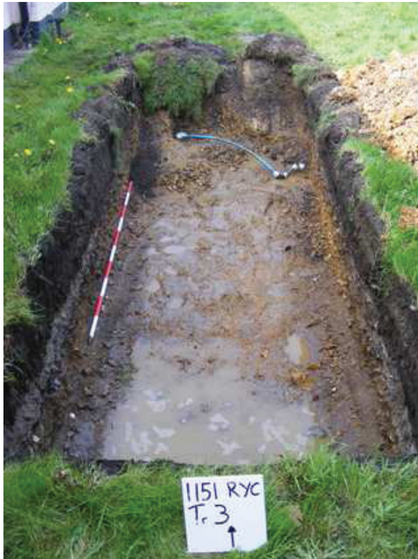
Plate 2: Trench 3 depicting the topsoil, made ground and natural geology of the site, and services
