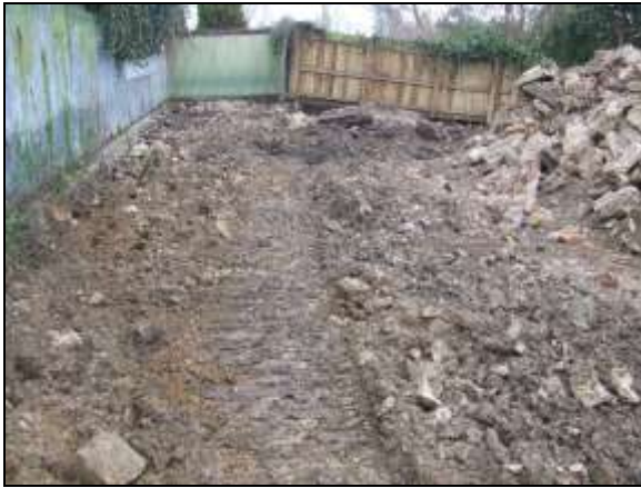
Plate 1: Concrete strip, facing southeast
