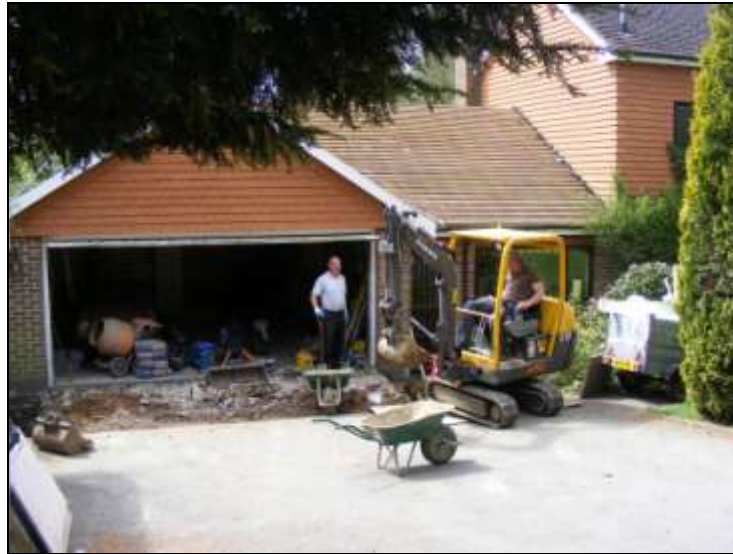
Plate 1: General working shot, looking south
