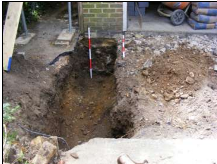
Plate 2: Eastern footing trench, looking south, 2x1m scales
