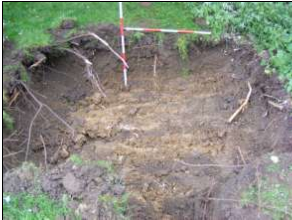
Plate 7: Soakaway, looking south.
