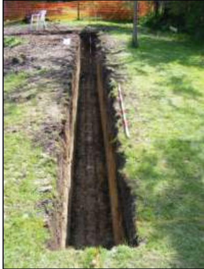
Plate 1: Footing trench, looking south
