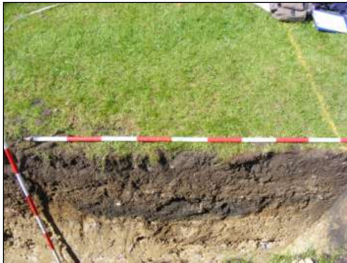
Plate 3: Pit [001] & Ditch [003] in footing trench, looking west.
