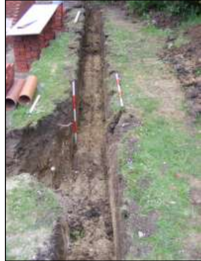
Plate 2: Service trench A, looking south.
