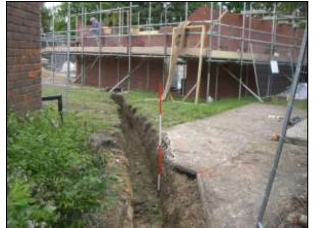
Plate 8: Service trench B looking south-west.
