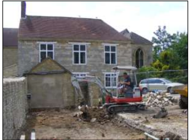
Plate 8: Overall ground reduction in progress, looking southwest
