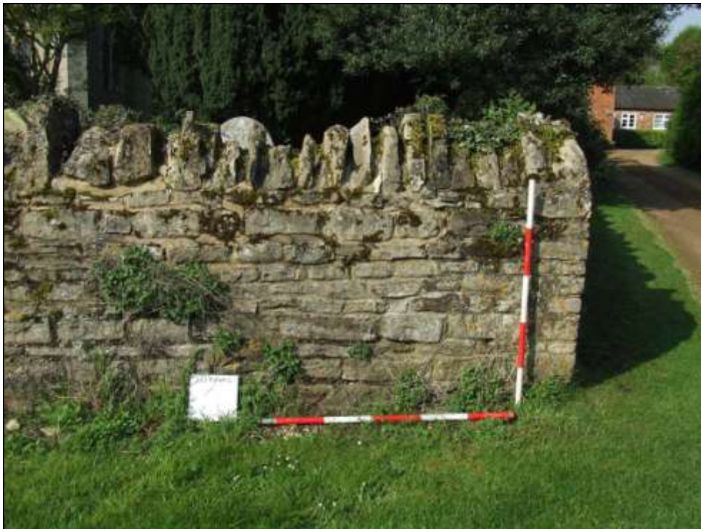
Plate 2: East facing side of boundary wall
