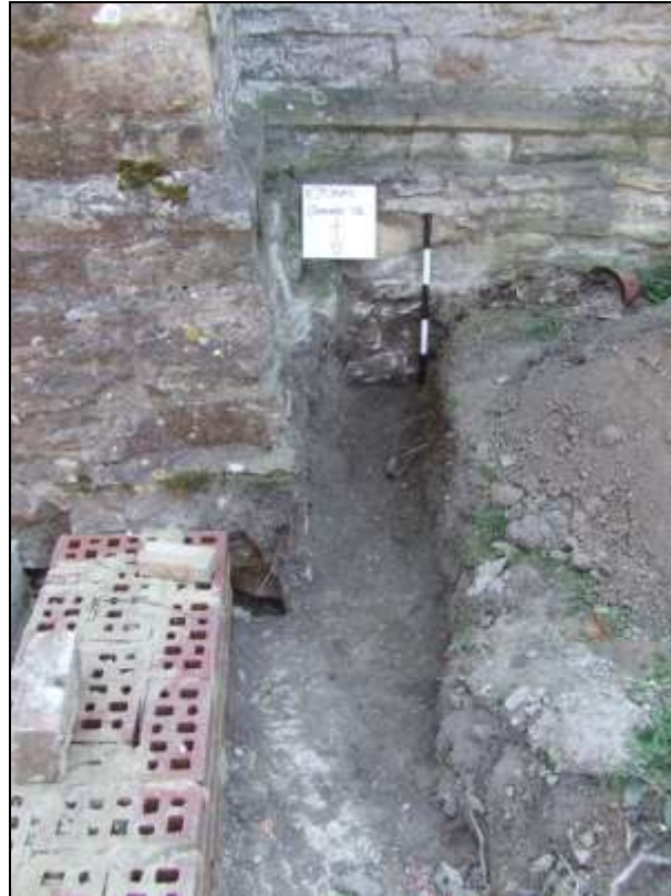
Plate 15: Drain 1 exposing north wall, looking South
