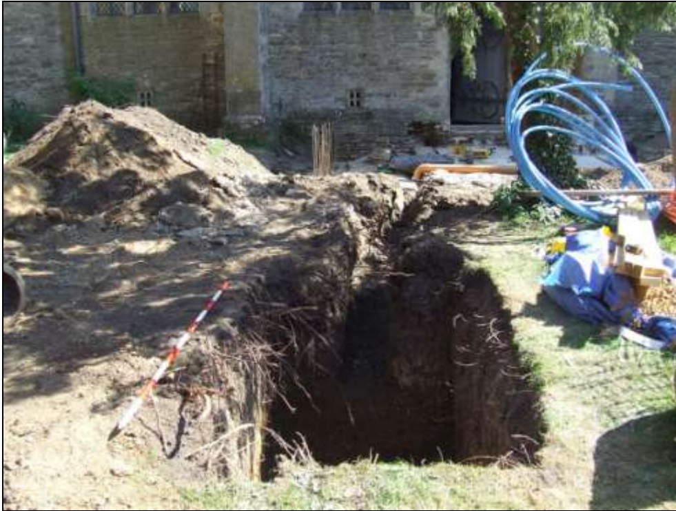
Plate 13: Soakaway and drains 1 and 2, looking South
