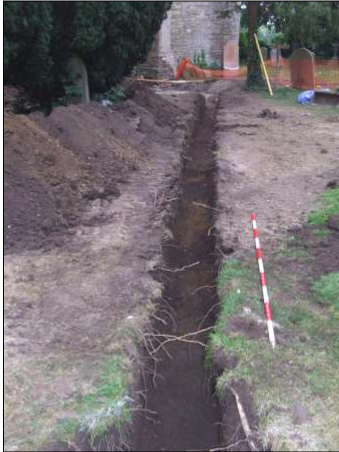
Plate 9: Main drainage trench between MH1 and MH2, looking SW
