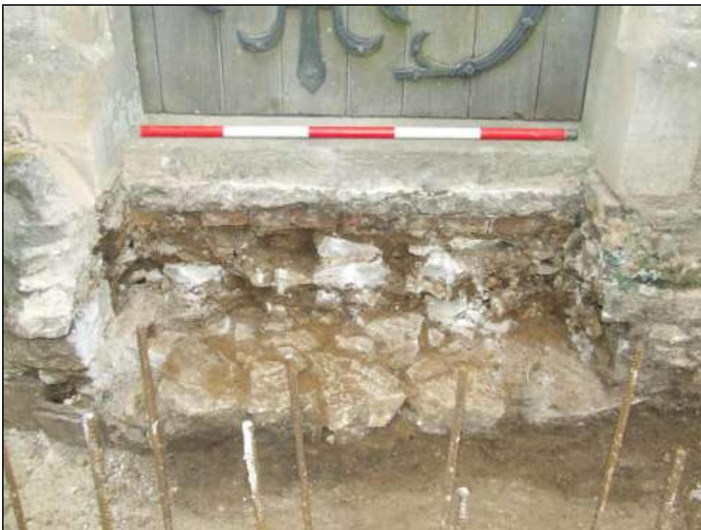
Plate 8: Exposed north wall beneath concrete step
