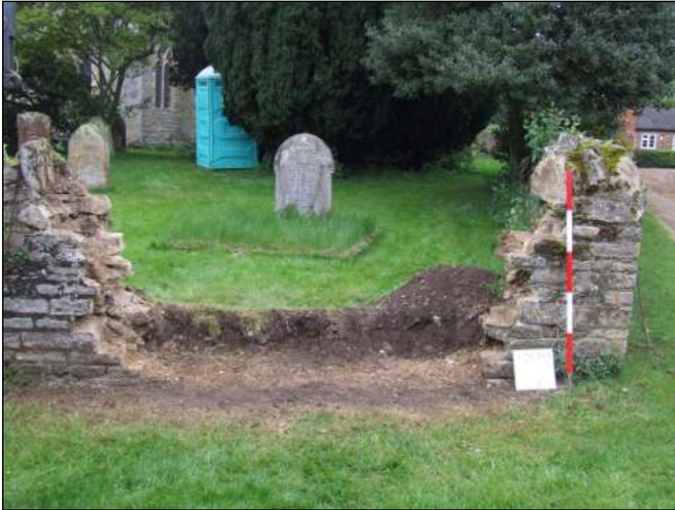
Plate 3: East facing side of boundary wall after demolition
