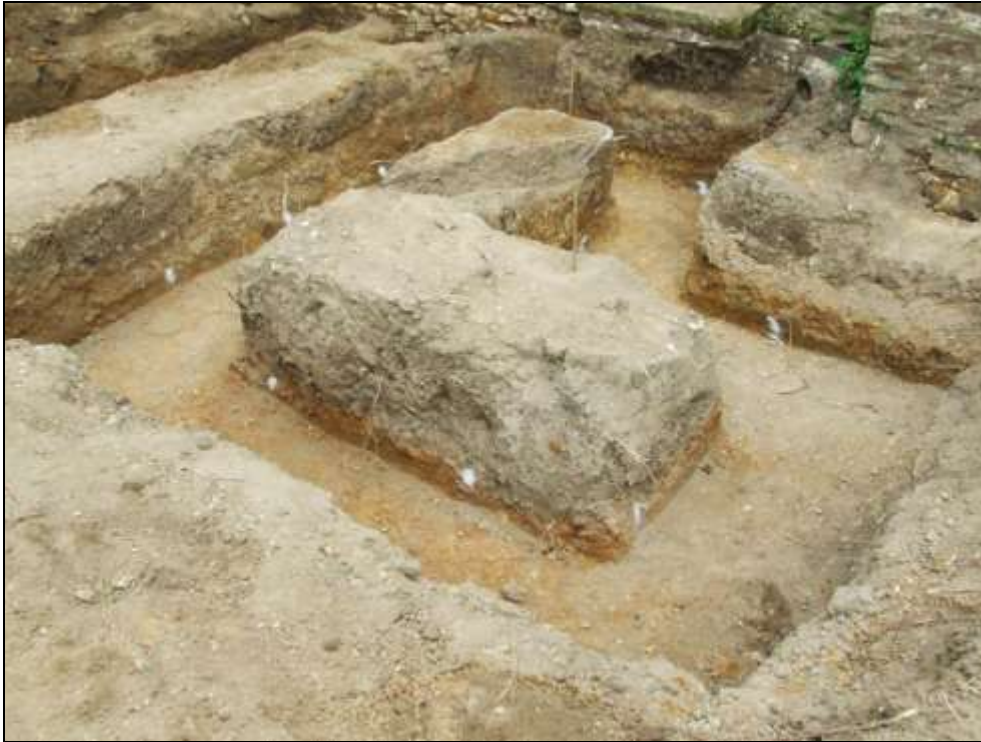
Plate 7: Footing trenches A and B, looking NW
