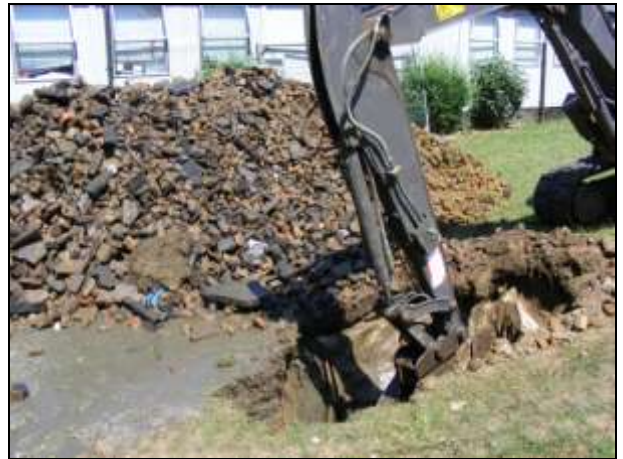
Plate 2: General shot of modern soakaway, looking east
