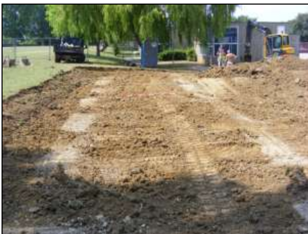
Plate 5: Overall ground reduction, looking northwest, 2m scale
