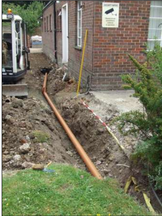
Plate 3: Foul drainage trench, looking east
