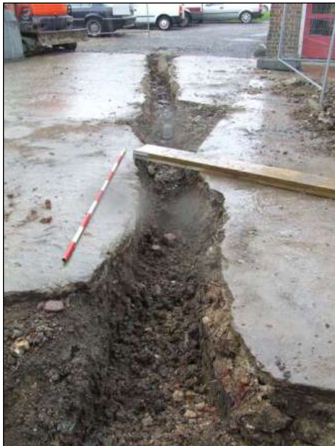
Plate 8: Drainage trench, looking west
