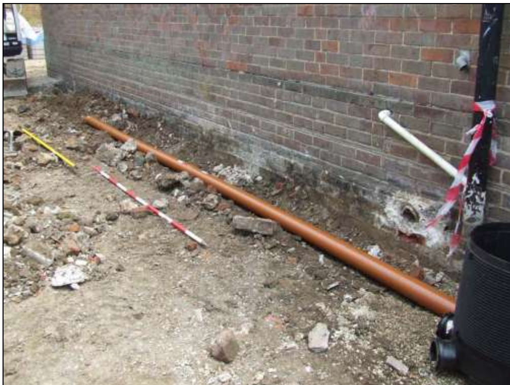
Plate 4: Foul drainage trench, looking southeast
