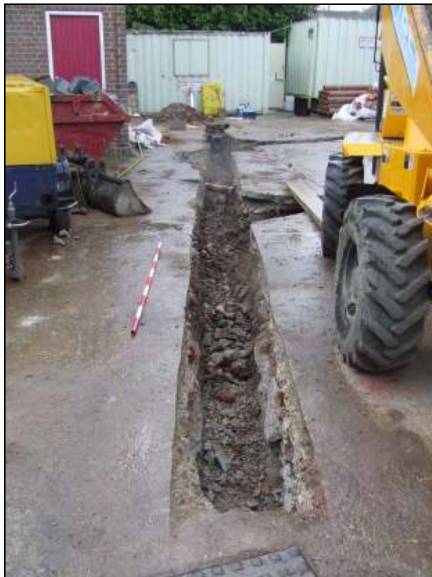
Plate 6: Drainage trench, looking southeast
