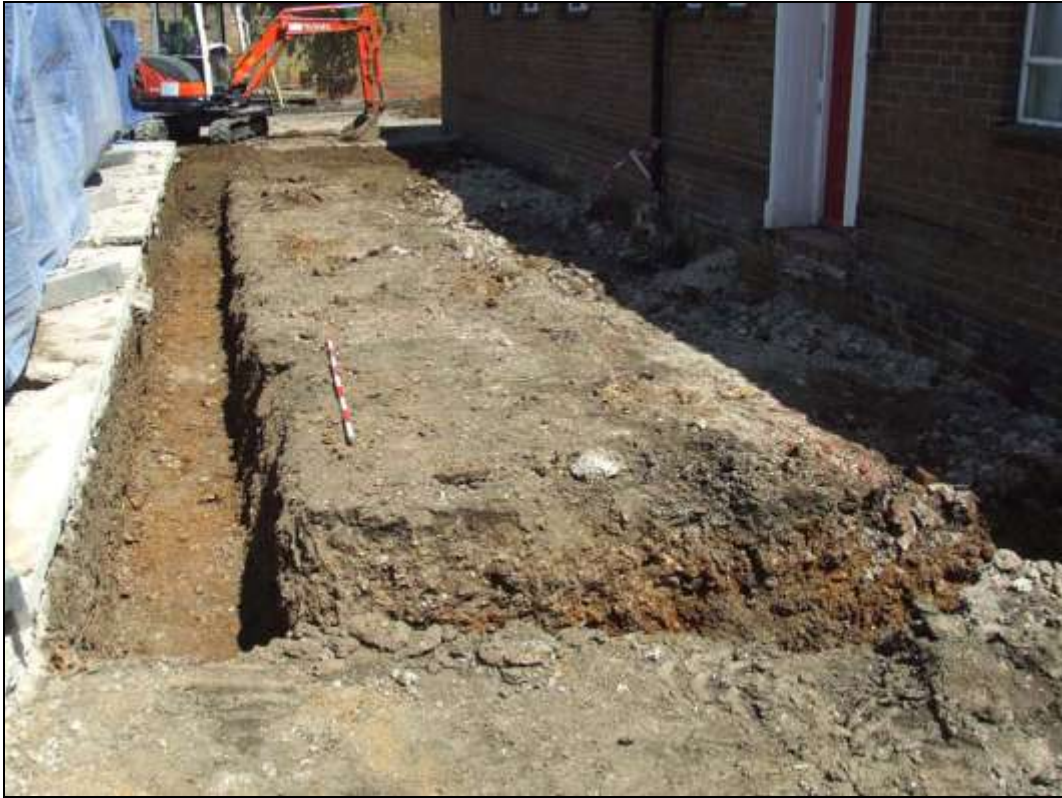
Plate 1: Development area and footing trench, looking east
