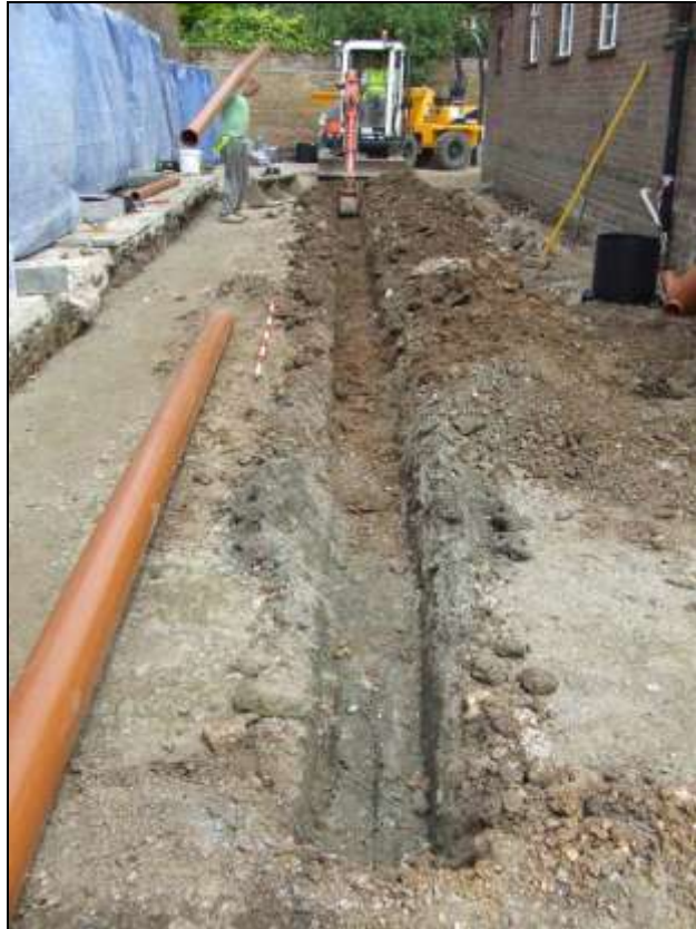
Plate 5: Storm drainage trench, looking east
