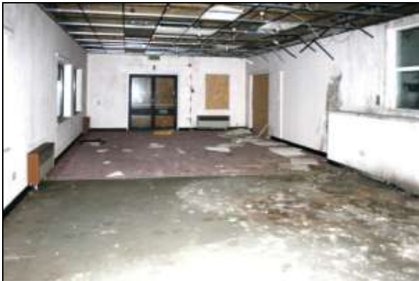
Plate 62: Building G, day room G18 looking south-west
