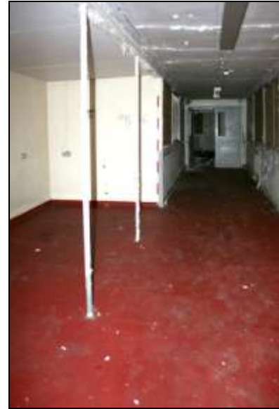
Plate 49: Building F, corridor F1 looking south-east
