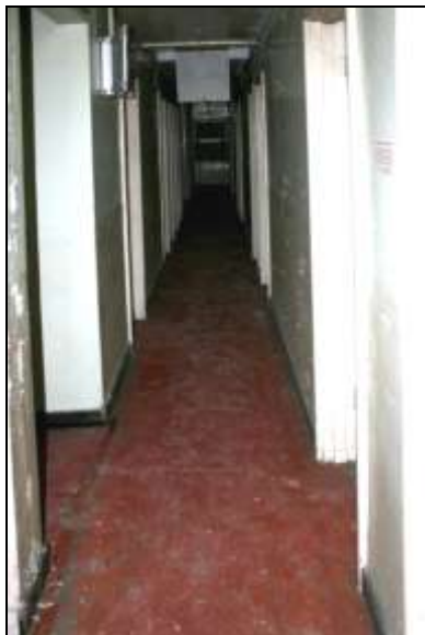
Plate 40: Building D, first floor, corridor D9 looking north-west
