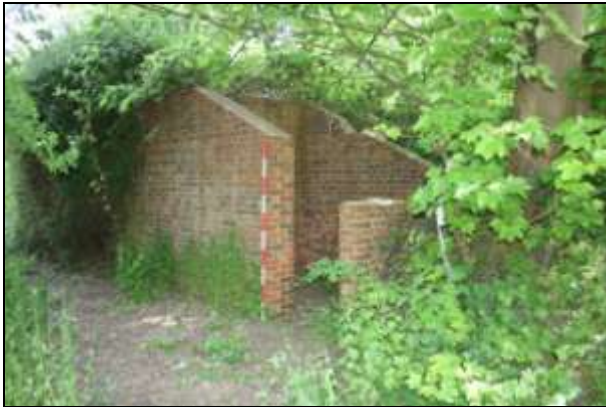
Plate 84: Building J, entrance from west
