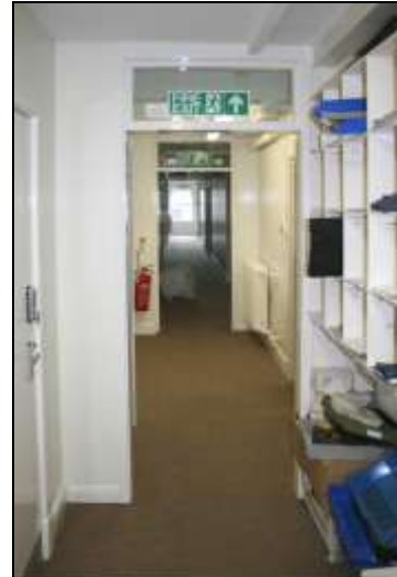
Plate 117: Building N first floor, corridor N9 looking south-east
