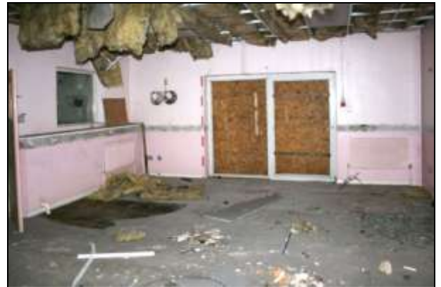
Plate 57: Building G, day room G7 looking north-east
