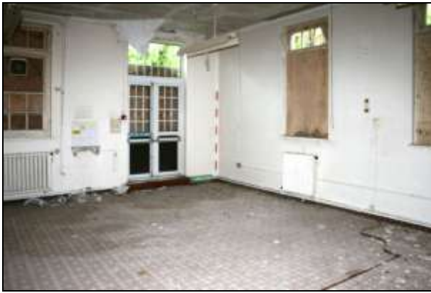
Plate 48: Building E, children's ward E7, looking south
