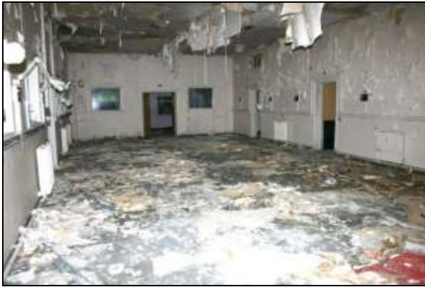
Plate 54: Building G, ward G4 looking north-west
