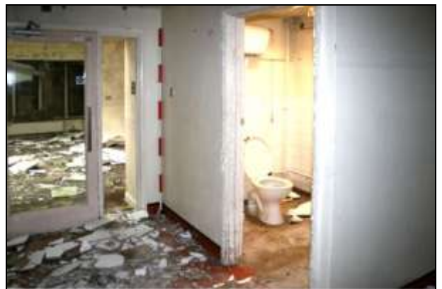
Plate 71: Building H, passage H19 and WC
