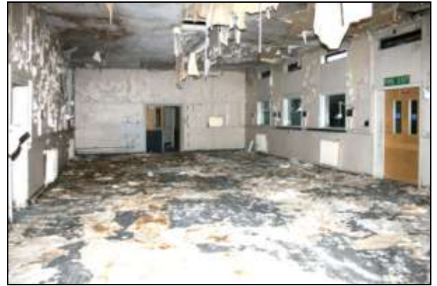
Plate 55: Building G, ward G4 looking south-east
