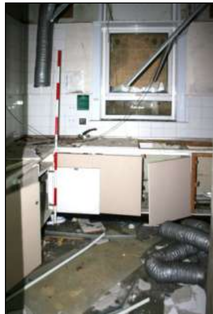
Plate 65: Building H, kitchen H2
