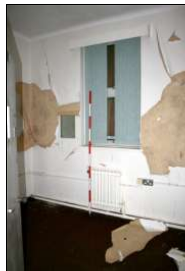
Plate 11: Building A ground floor, private room A20, looking south
