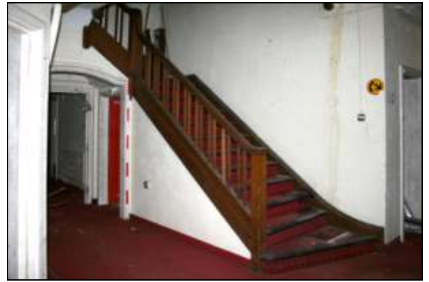
Plate 13: Building A ground floor A1, stairs looking east
