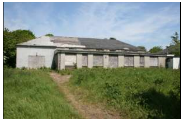
Plate 53: Building G, south-west elevation
