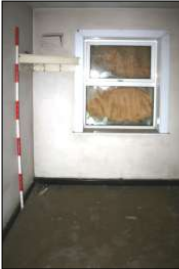
Plate 42: Building D, first floor, bedroom D10 looking north-east
