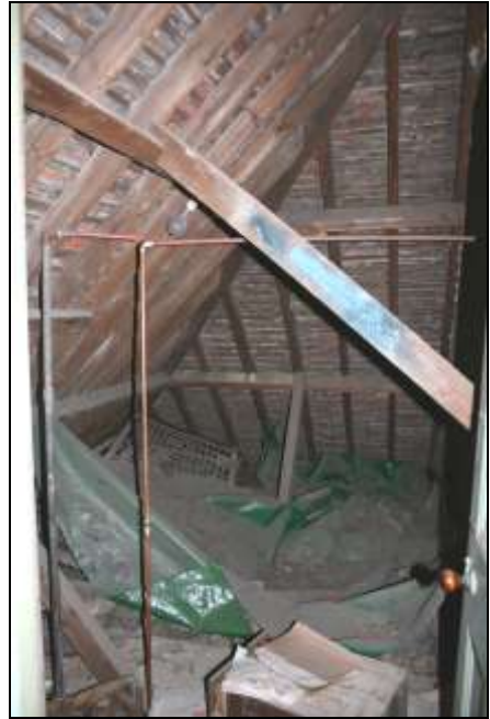
Plate 133: Building O attic, rear roof space looking north-west
