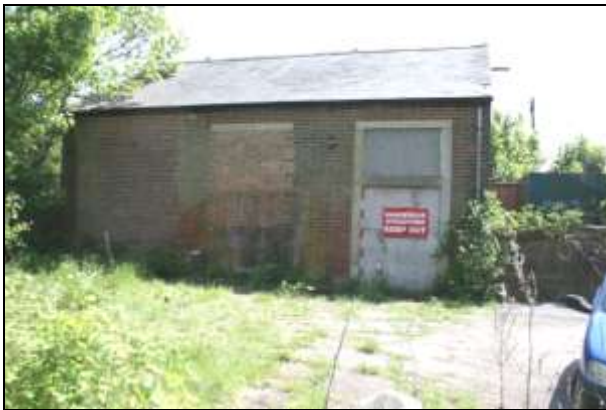
Plate 92: Building K, north-west elevation
