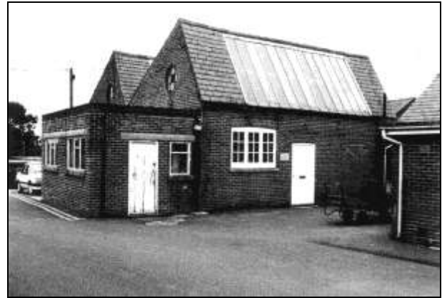
Plate 91: Building K from east
