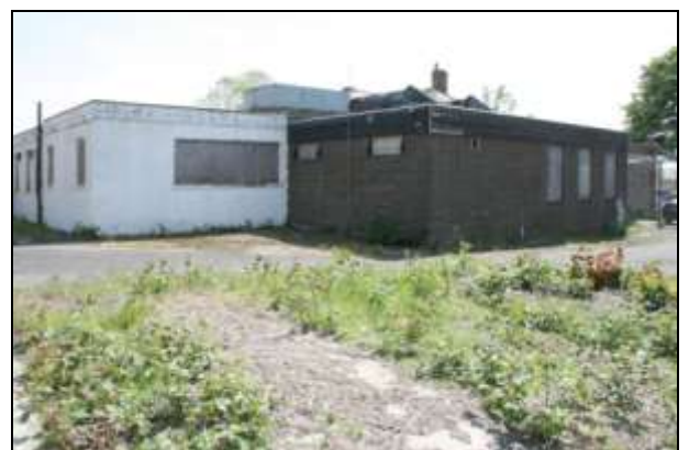
Plate 17: Building B, theatre block, north-west elevation
