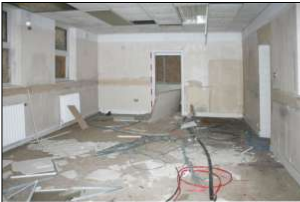
Plate 38: Building D, nurses' dining room D7, looking south-east
