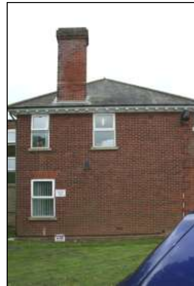
Plate 109: Building N, north-east elevation, west end
