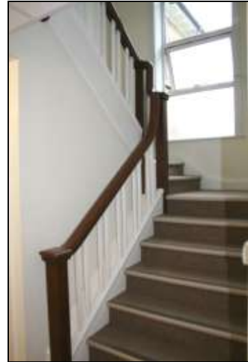
Plate 115: Building N ground floor, north-west stairs
