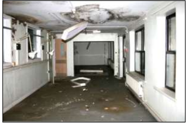
Plate 61: Building G, ward extension G16 looking south-east
