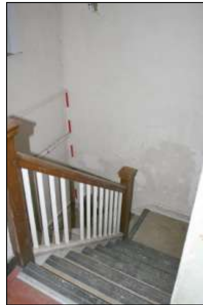
Plate 39: Building D, first floor, south-east stairs
