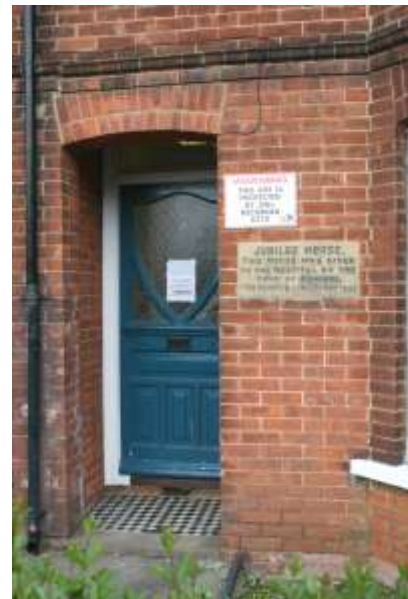
Plate 123: Building O, south-east elevation, detail of front door
