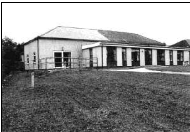
Plate 52: Building G, south-west elevation
