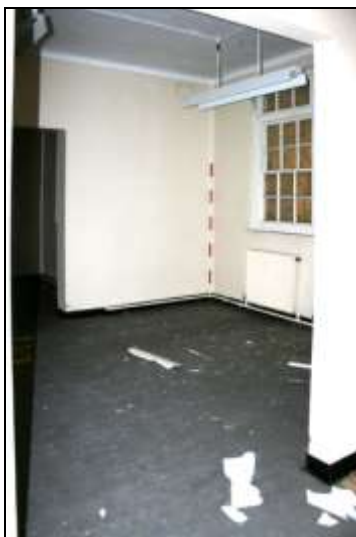
Plate 46: Building E, labour ward E5, looking north-west
