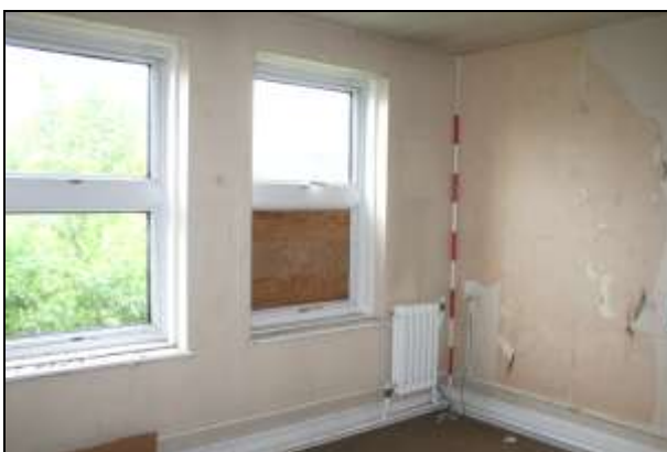
Plate 16: Building A first floor, Room A30 looking east
