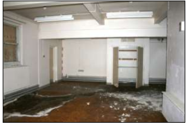
Plate 19: Building B, recovery room? B1, looking south-east
