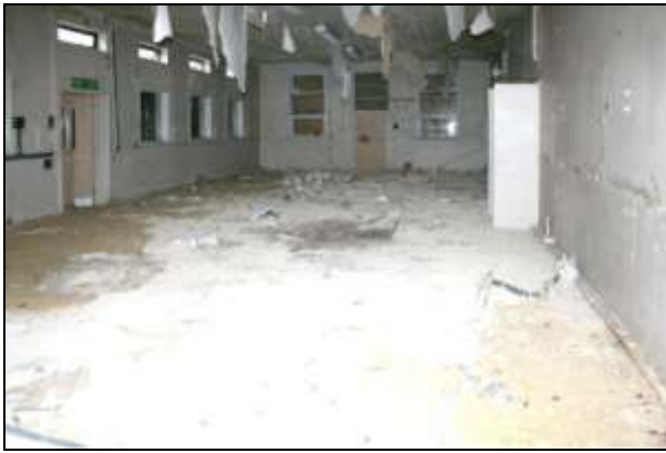
Plate 66: Building H, Ward H4 looking south-east
