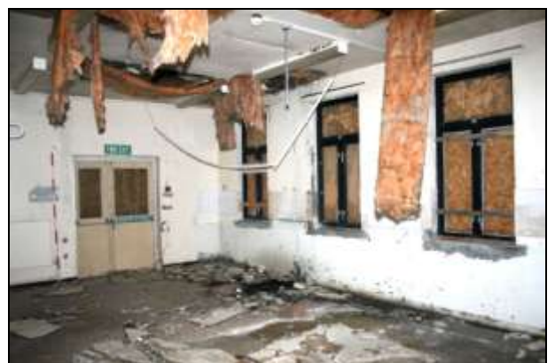
Plate 23: Building B, Room B6, looking west
