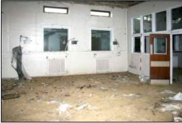
Plate 60: Building G, ward G14 looking west
