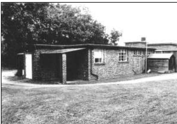
Plate 100: Building M, from south
