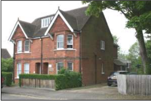
Plate 120: Building O, south-east elevation from east
