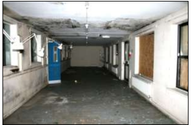
Plate 69: Building H, extension H5 looking south-east
