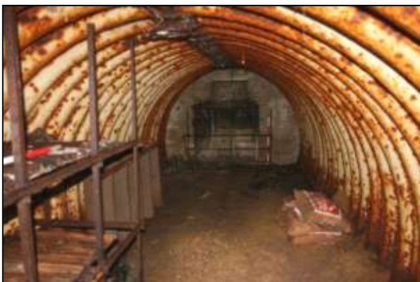
Plate 88: Building J, interior looking south-east
