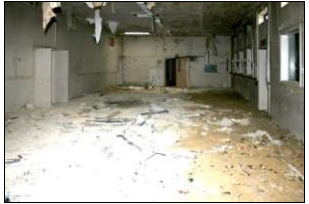
Plate 67: Building H, ward H4 looking north-west
