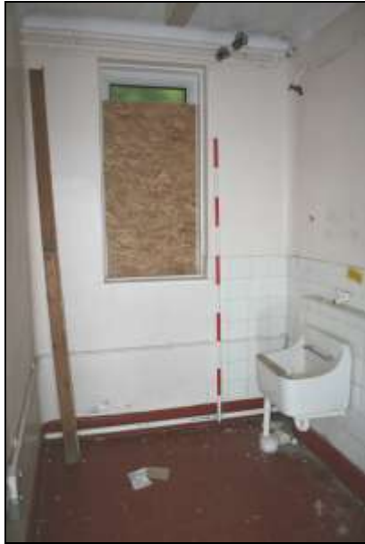
Plate 12: Building A ground floor, sluice A23, looking east
