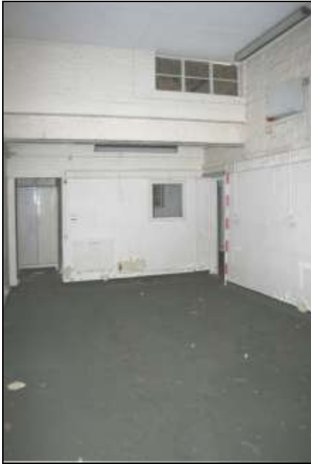
Plate 102: Building M, treatment room M2 looking south-east
