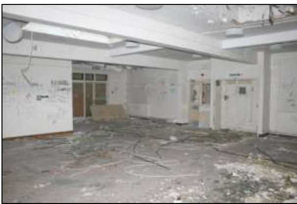
Plate 32: Building C, reception C8, looking east
