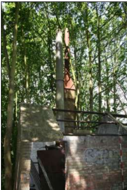
Plate 134: Building P, close-up from south-west
