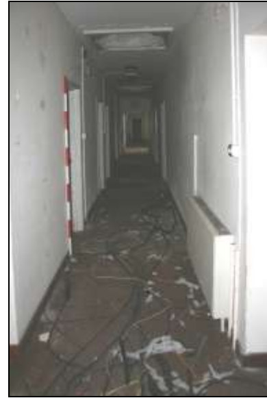
Plate 79: Building I, corridor I3, looking south-west
