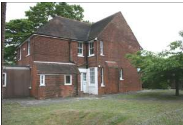
Plate 122: Building O, south-west elevation
