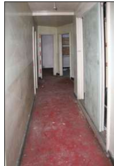
Plate 41: Building D, first floor, corridor to D11 looking south-west
