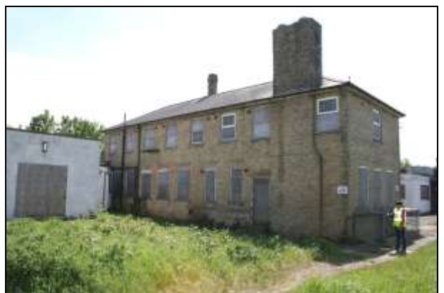
Plate 35: Building D, north-east elevation
