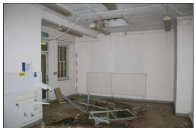
Plate 29: Building C, Room C5 looking south
