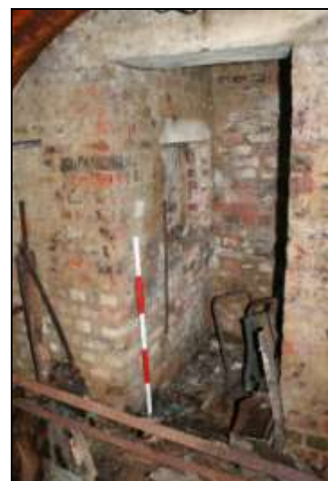
Plate 89: Building J, escape hatch and south-east compartment
