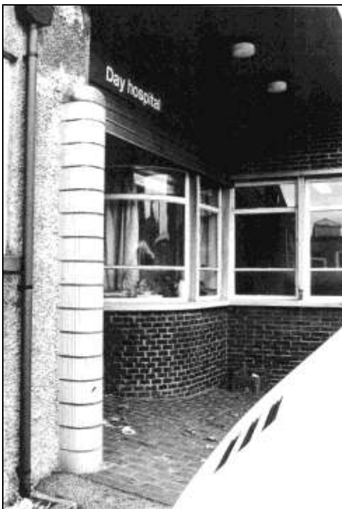
Plate 74: Building I, north-west entrance
