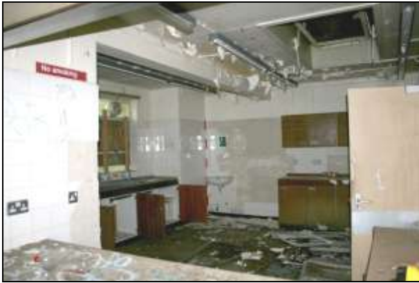
Plate 30: Building C, kitchen? C6, looking west
