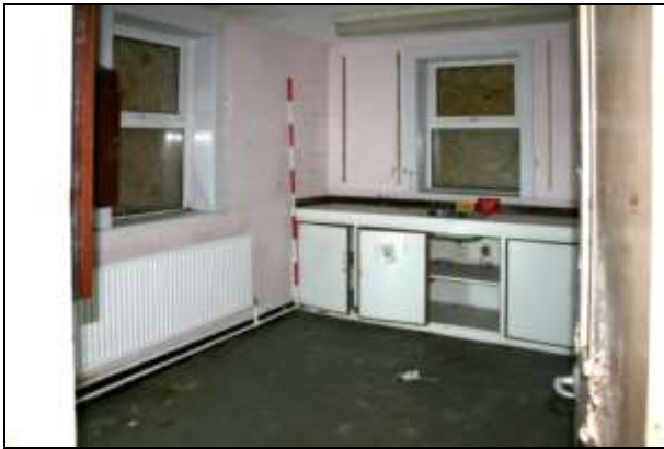
Plate 68: Building H, dispensary H7
