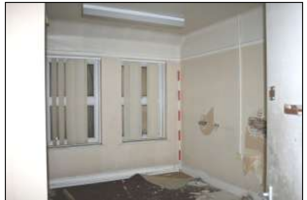
Plate 15: Building A first floor, house surgeon's sitting room A32, looking west
