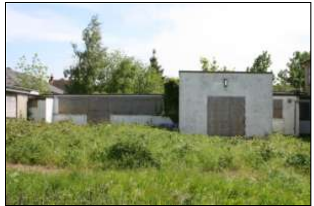
Plate 81: Building C/E corridor, north-west elevation
