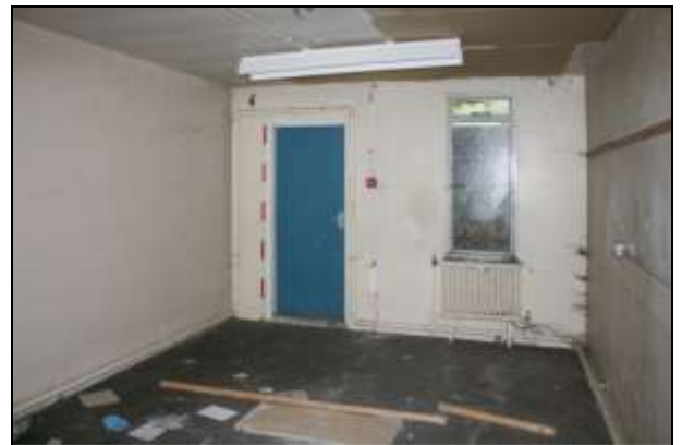
Plate 51: Building F, storeroom F3, looking south-west
