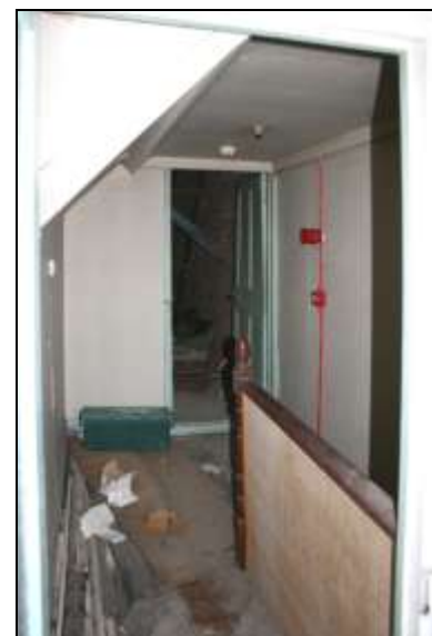
Plate 131: Building O attic, landing O16 looking north-west
