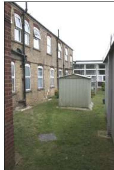
Plate 111: Building N, south-east elevation, looking east
