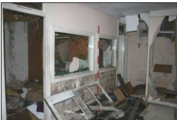
Plate 94: Building K, laundry interior
