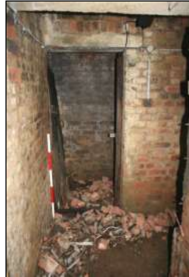
Plate 85: Building J, entrance lobby and toilet doorway
