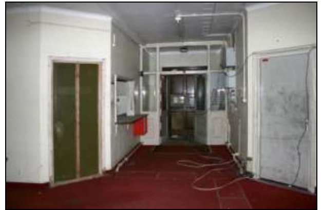
Plate 7: Building A ground floor, foyer A1, looking north-west
