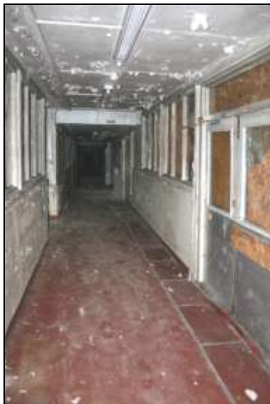
Plate 82: Building G/F corridor, looking south-west
