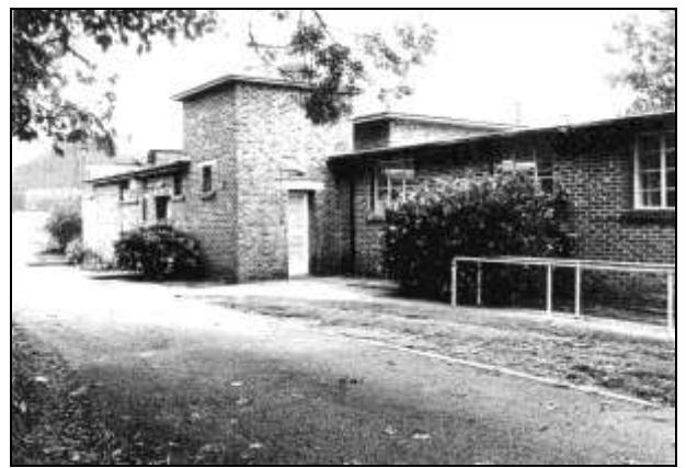
Plate 101: Building M, from west
