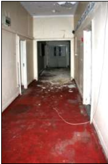
Plate 44: Building E, corridor E1 looking north-west
