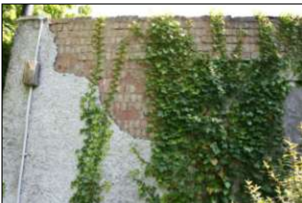
Plate 64: Building H, north-west elevation, detail of brickwork
