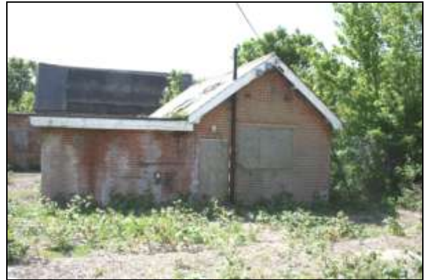
Plate 97: Building L, north-east elevation
