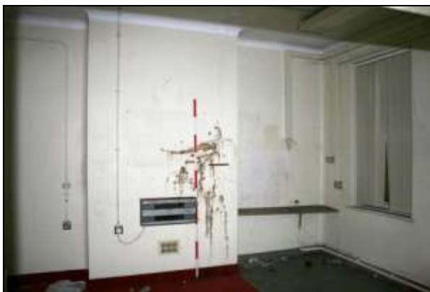
Plate 10: Building A ground floor, main office A5 looking south-east
