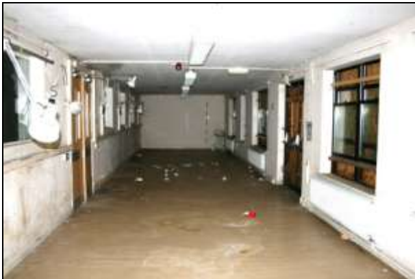
Plate 56: Building G, ward extension G5 looking south-east
