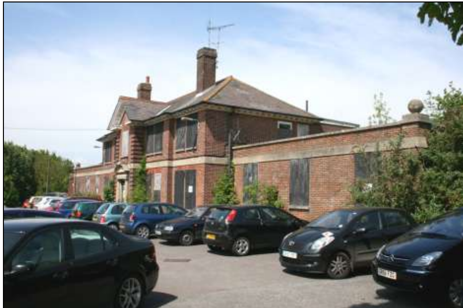
Plate 5: Building A, general view from south-east
