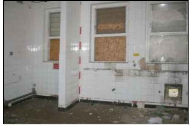
Plate 37: Building D, scullery D3 looking south-west
