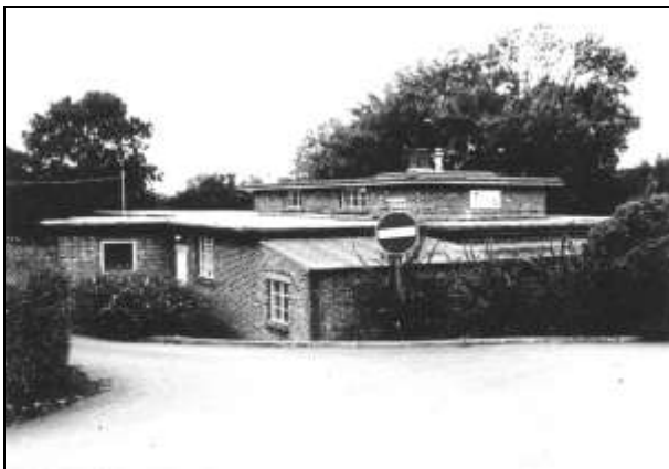
Plate 98: Building M, from north-east
