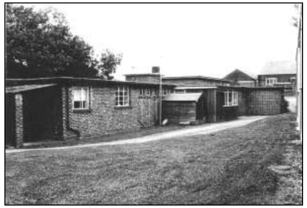
Plate 99: Building M, from south
