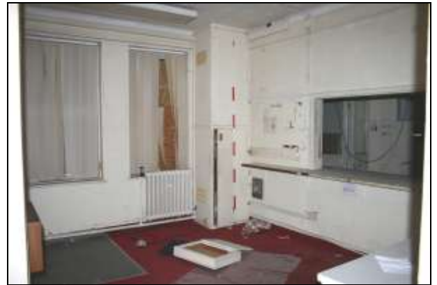
Plate 9: Building A ground floor, main office A5 looking west
