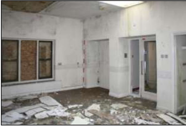
Plate 72 Building H, day room H20 looking south
