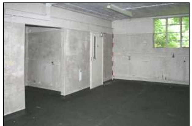
Plate 107: Building M, Room M9 looking east
