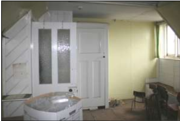
Plate 132: Building O attic, room O17 looking east
