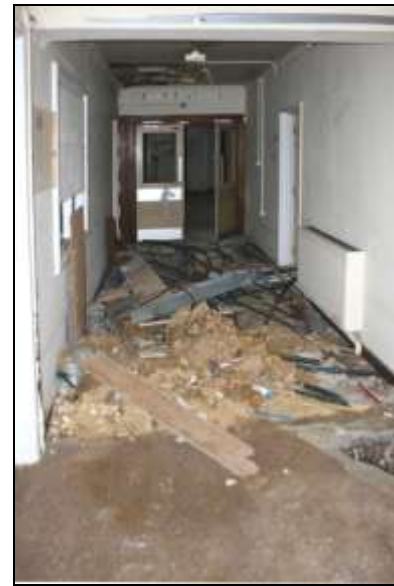
Plate 25: Building C, corridor C1 looking south-east
