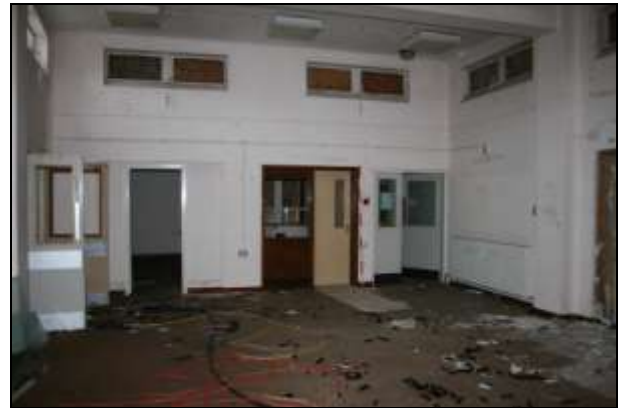
Plate 75: Building I, lobby I4 looking south-west
