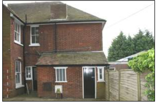
Plate 121: Building O, north-east elevation
