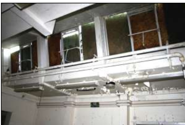
Plate 22: Building B, theatre B5, detail of roof lights
