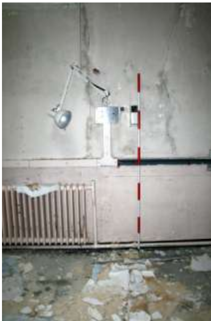
Plate 70: Building H, ward H15, surviving fittings at bed location
