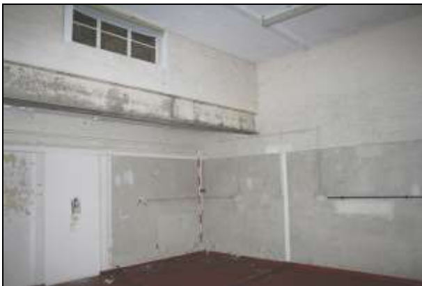
Plate 104: Building M, gym M6, looking north
