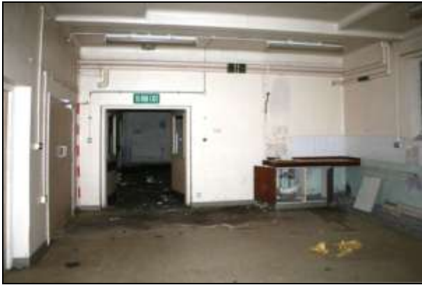
Plate 18: Building B, theatre B2, looking south-west
