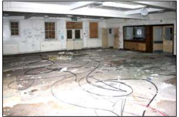
Plate 31: Building C, reception C8, looking west
