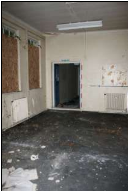
Plate 50: Building F, ward F2, looking south-west
