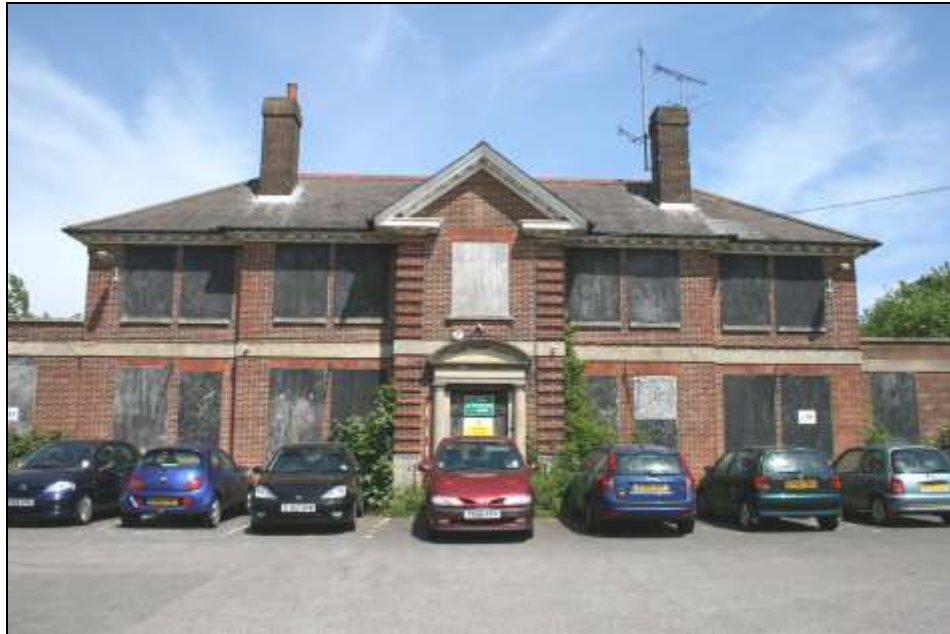
Plate 4: Building A, south-west elevation
