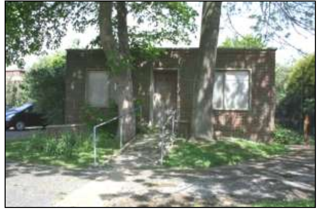
Plate 73: Building I, south-west elevation
