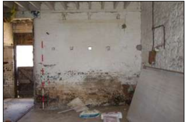
Plate 10: Building 1, Area 1a, looking north, 2m scale
