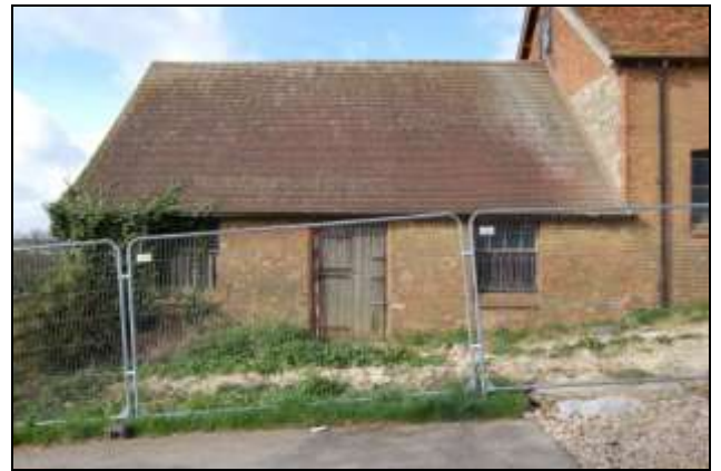
Plate 4: Building 2, north elevation, 2m scale
