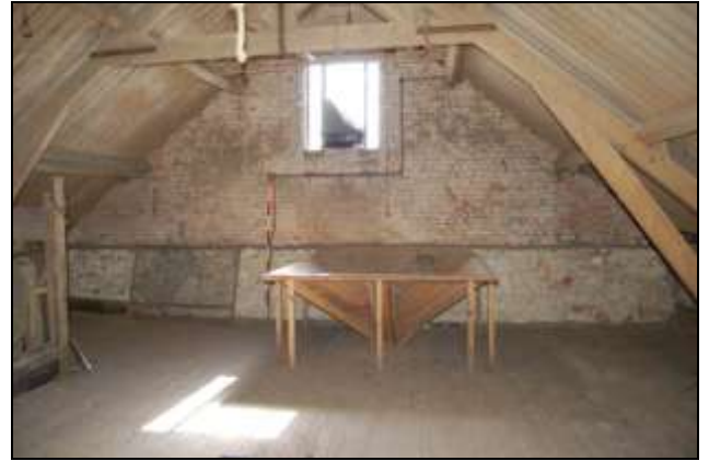
Plate 14: Building 1, grain store, looking east, 2m scale
