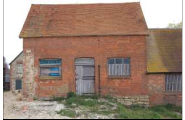
Plate 2: Building 1, south elevation, 2m scale
