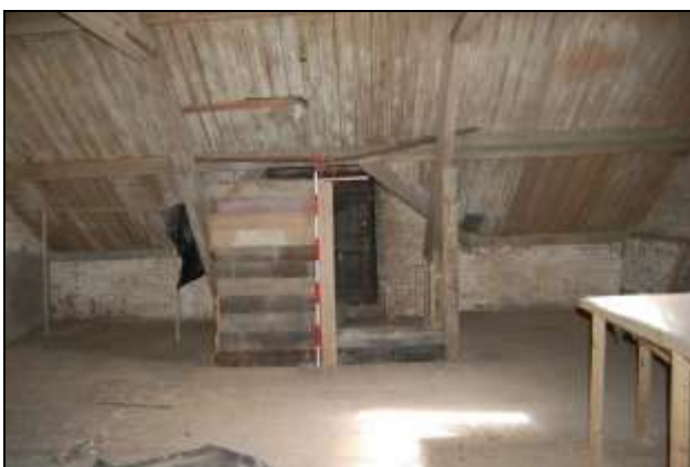
Plate 17: Building 1, grain store, looking north, 2m scale
