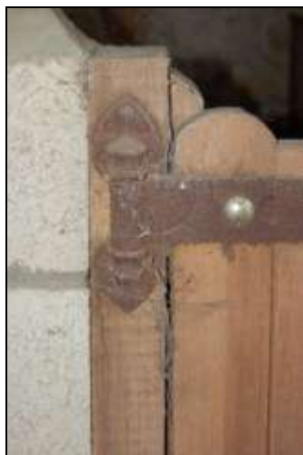
Plate 23: Building 2, detail of decorative hinges on doors in west wall
