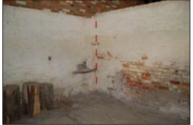
Plate 20: Building 2, Area 2b, looking south east, 2m scale
