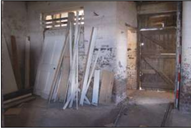
Plate 7: Building 1, Area 1a, looking north west, 2m scale
