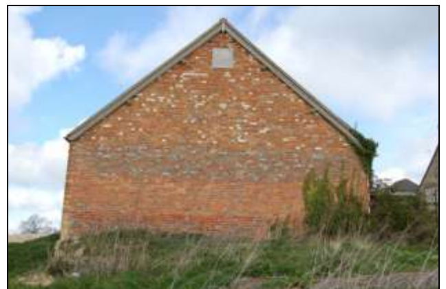
Plate 6: Building 2, west elevation, 2m scale
