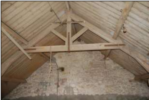
Plate 15: Building 1, grain store, roof truss, looking west, 2m scale
