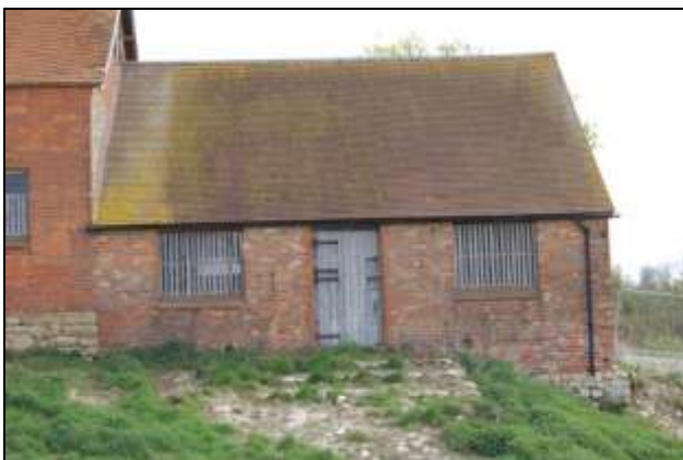
Plate 5: Building 2, south elevation
