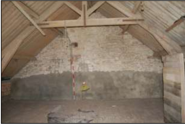
Plate 13: Building 1, grain store, looking west, 2m scale
