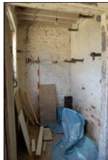
Plate 12: Building 1, Area 1c, looking east, 2m scale
