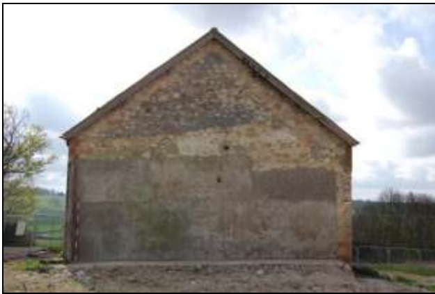
Plate 3: Building 1, west elevation, 2m scale
