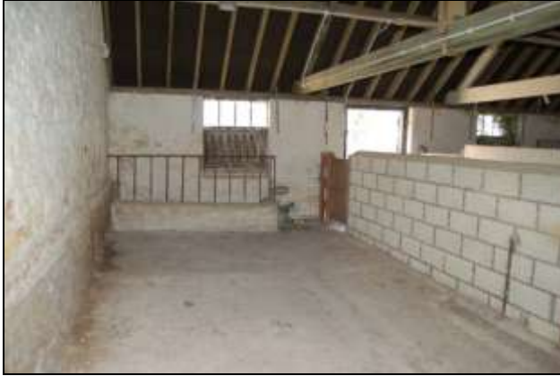
Plate 19: Building 2, Area 2a, looking north, 2m scale
