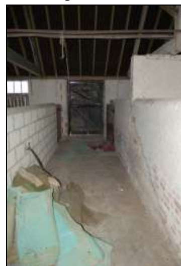
Plate 18: Building 2, looking south, 2m scale
