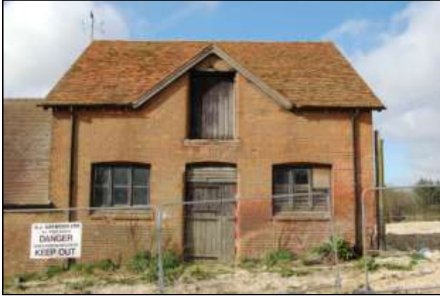
Plate 1: Building 1, north elevation, 2m scale
