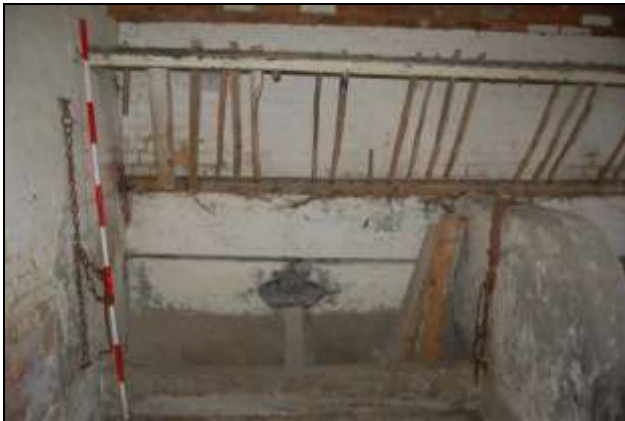
Plate 21: Building 2, Area 2c, looking east, 2m scale
