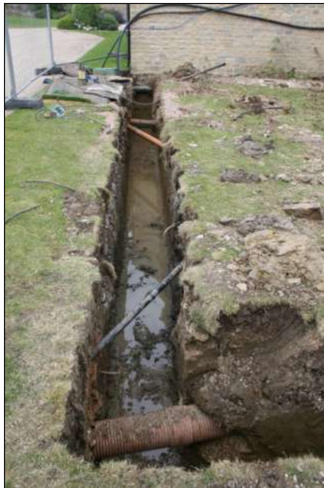
Plate 3: South footing trench, showing modern services present
