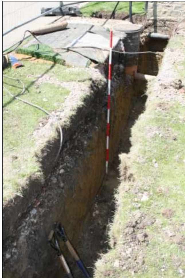
Plate 1: South footing trench, north-facing section
