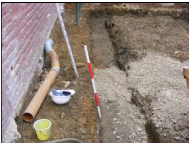
Plate 5: Footing trench easterly run, looking southwest, 1 metre scale.
