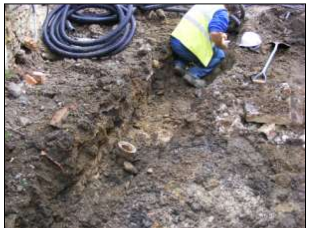
Plate 6: Service trench looking northeast.
