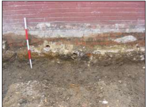
Plate 4: Footing trench southerly run, looking southwest, 1 metre scale.
