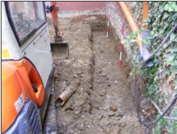
Plate 3: Footing trench westerly run, looking southwest, 2x1 metre scale.
