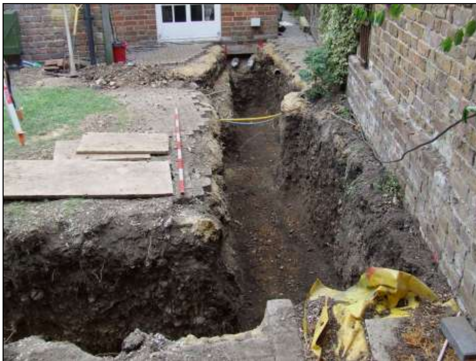
Plate 3: Northwest area of footing trench, looking west
