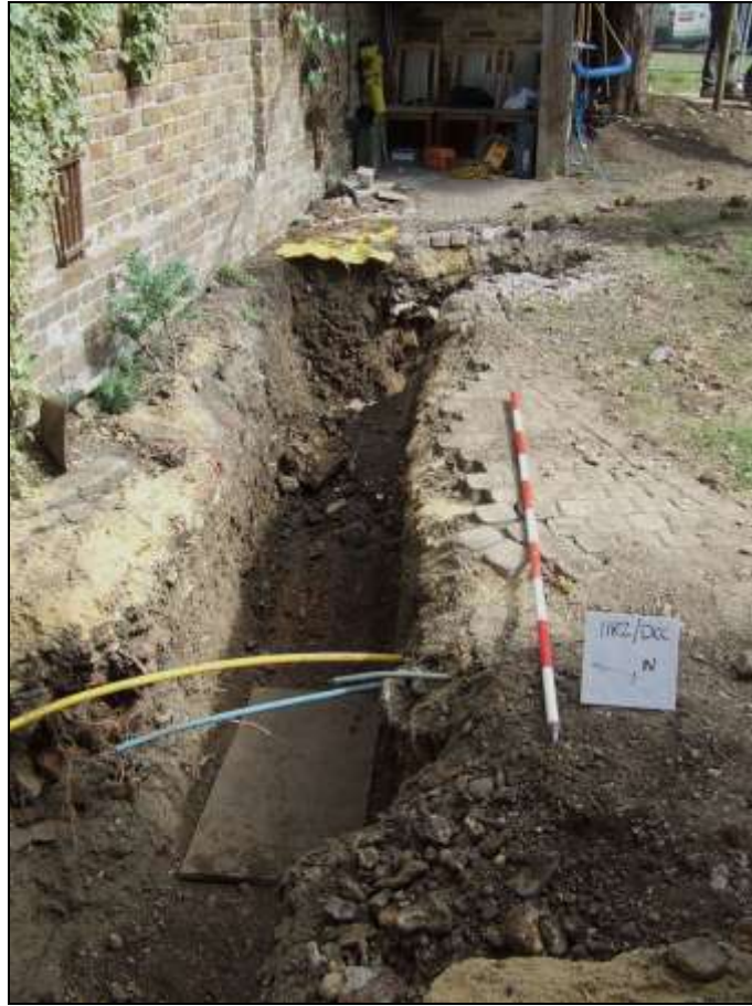
Plate 2: Northwest area of footing trench, looking east
