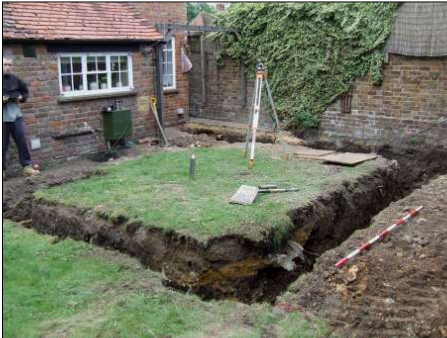
Plate 1: Overall footing trench, looking NW
