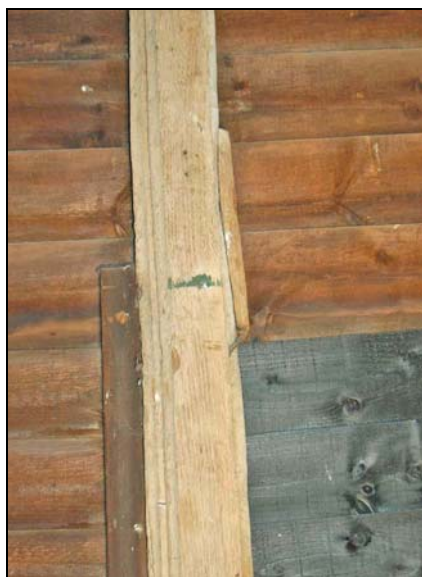
Plate 17: Hollow chamfer moulding on stud
