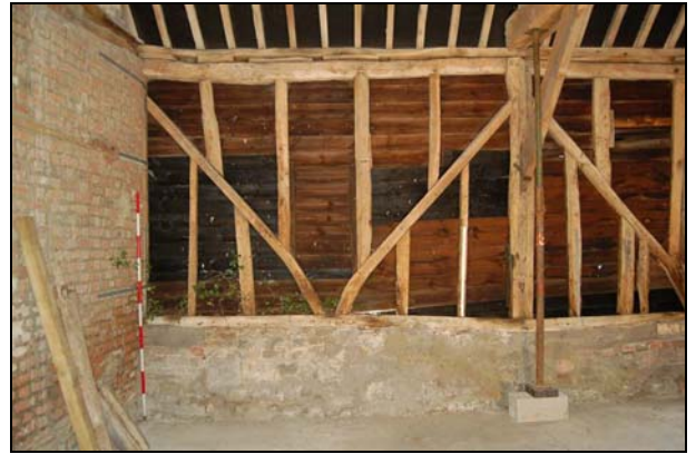
Plate 14: East wall: Bay 3
