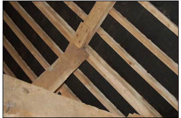
Plate 20: Simple splayed scarf joint
