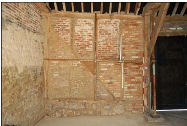
Plate 11: West wall: Bay 3
