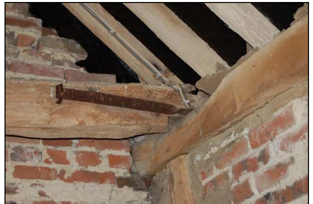
Plate 22: Iron tie & new rafters
