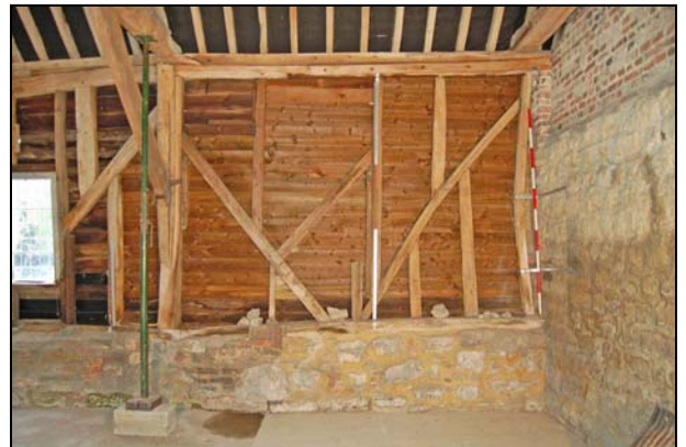
Plate 16: East wall: Bay 1
