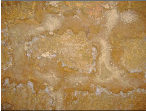
Plate 7: Mortared Whitchurch Sandstone
