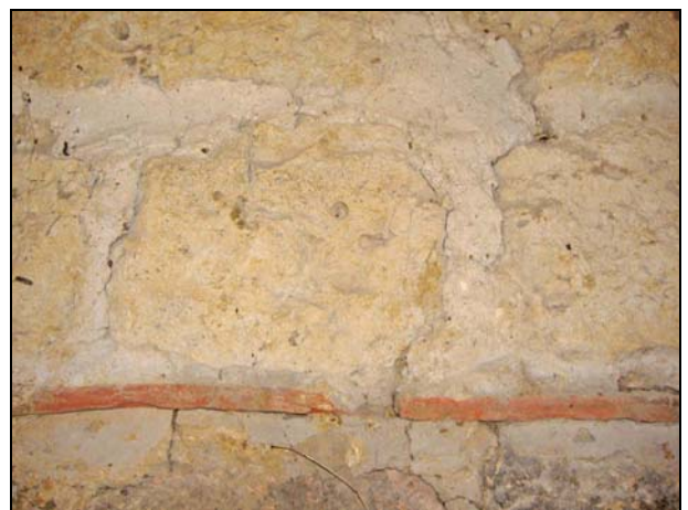
Plate 6: Interior stone work detail
