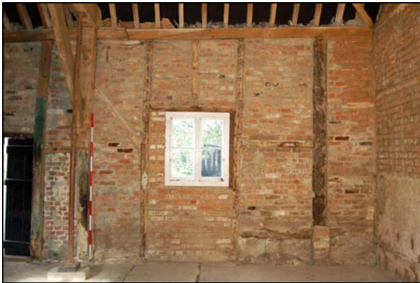
Plate 9: West wall: Bay 1
