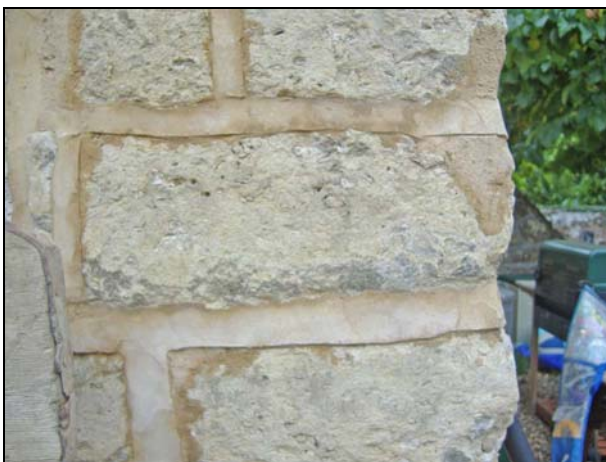
Plate 5: Ashlared Portland Limestone detail
