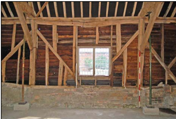
Plate 15: East wall: Bay 2
