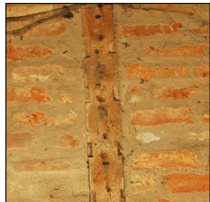
Plate 12: Re-used joist
