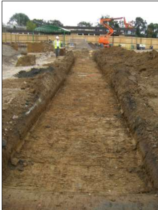
Plate 3: Overall view of trench 3 looking east
