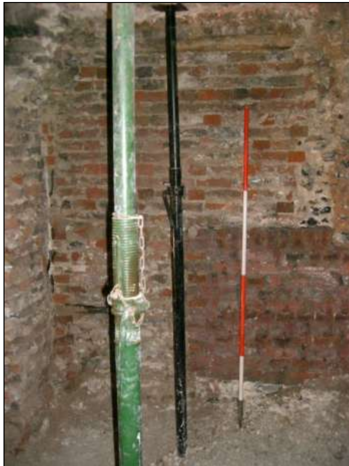
Plate 2: East facing brick elevation
