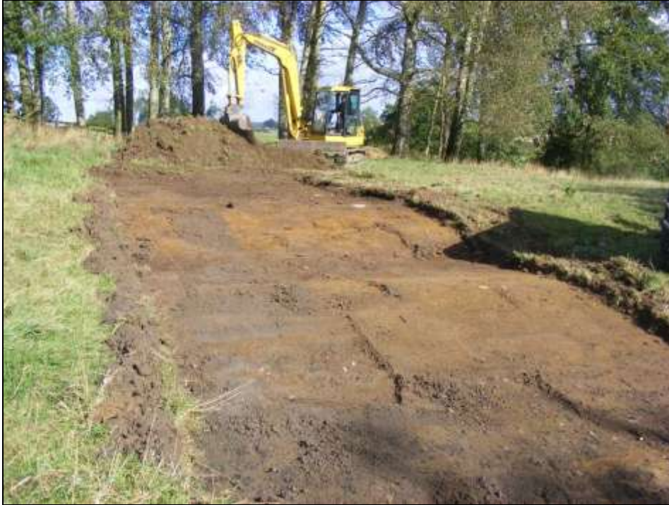
Plate 1: General view of site stripping, looking northwest
