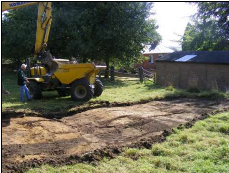
Plate 2: Working shot showing area partially stripped, looking east
