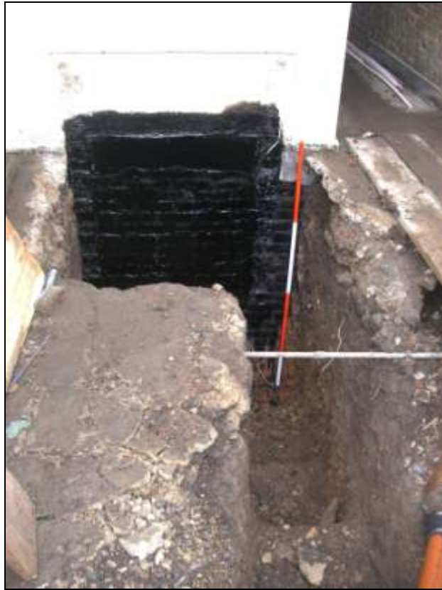
Plate 1: Footing and blocked cellar window, from east
