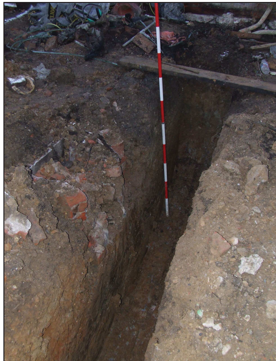
Plate 2: Footing trench F2, looking northwest, 2m scale
