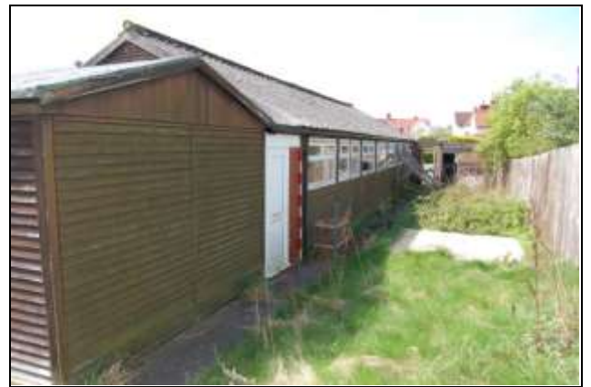
Plate 4: Memorial Hall, north elevation, 2m scale
