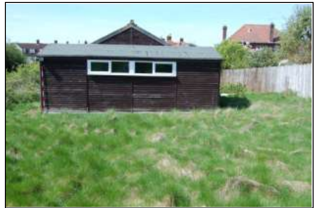
Plate 2: Memorial Hall, west elevation, 2m scale
