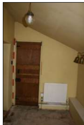
Plate 12: G1, looking south, 2m scale
