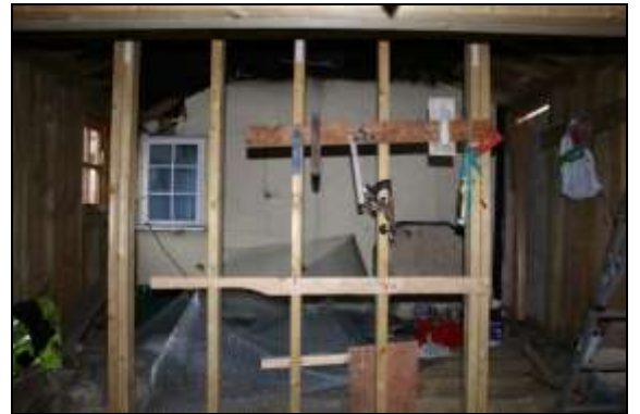
Plate 10: East end of north elevation, within new extension
