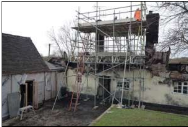
Plate 3: North elevation, showing full height of chimney stacks prior to removal
