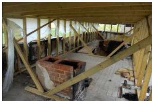
Plate 36: First floor looking west
