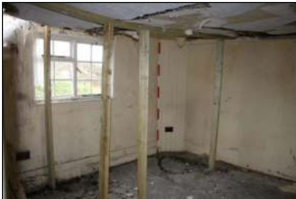
Plate 15: G2, looking north east, 2m scale
