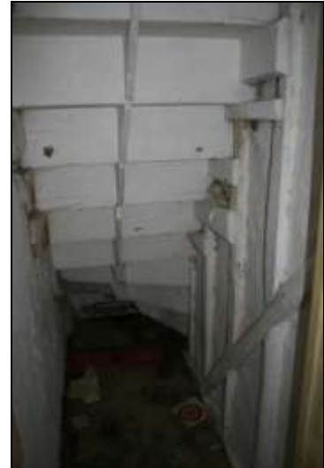
Plate 14: Cupboard under stairs in G1a, looking north
