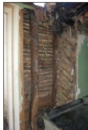
Plate 30: Exposed pole and diagonal laths in northwest corner of G4
