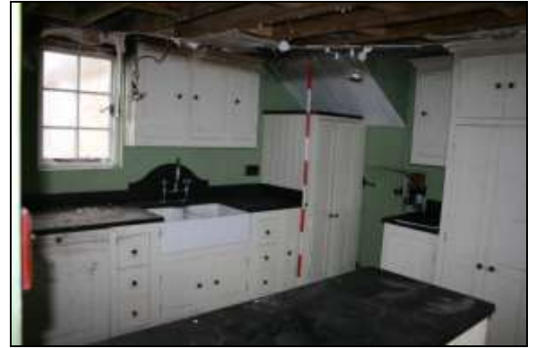
Plate 26: G4, looking north east, 2m scale
