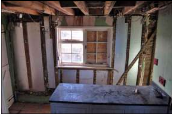
Plate 25: G4, looking south, after removal of plaster 2m scale
