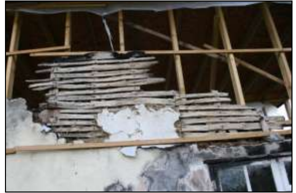
Plate 8: Exposed area of original construction material in north elevation
