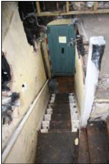
Plate 33: G5, looking south, 2m scale
