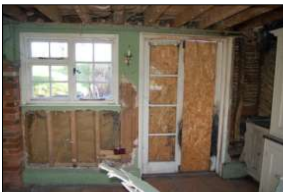
Plate 23: G3, looking north, 2m scale
