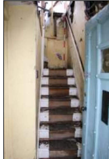
Plate 32: G5, looking north, 2m scale
