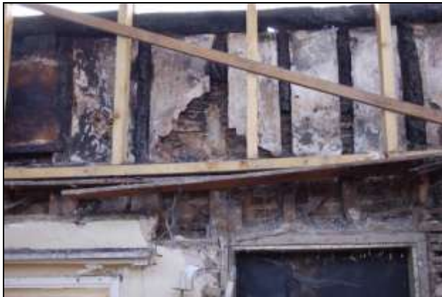
Plate 39: Example of first floor studwork in the south wall
