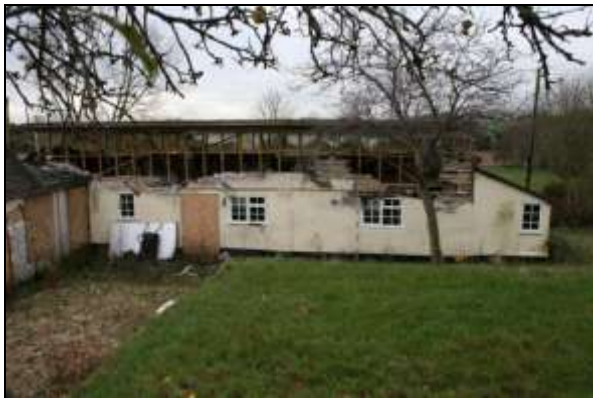
Plate 9: North elevation, 2m scale
