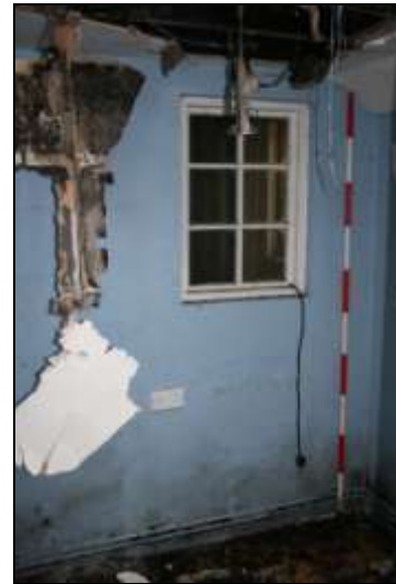
Plate 34: G6, looking north, 2m scale
