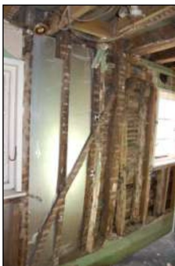
Plate 29: Passageway between G3 and G4, after removal of plaster
