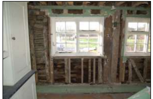
Plate 22: G3, looking south, 2m scale
