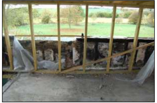
Plate 38: First floor, south wall
