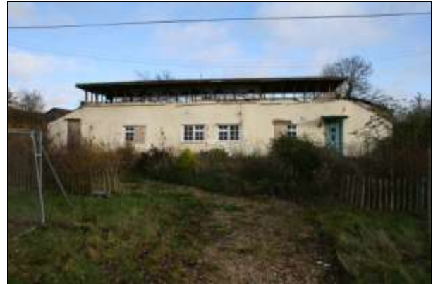
Plate 2: South elevation after the fire
