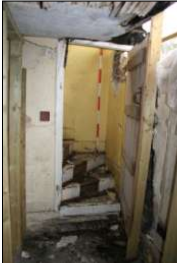
Plate 19: Stairs in northwest corner of G2, looking west, 2m scale
