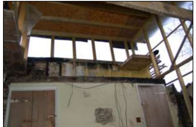
Plate 40: Studwork in west wall
