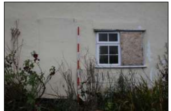
Plate 6: Blocked doorway in south elevation, looking north, 2m scale
