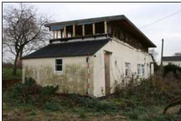
Plate 5: South and west elevations showing modern stable door, 2m scale
