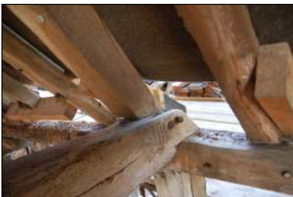
Plate 17: Carpenters assembly marks on Truss 1
