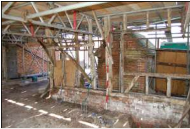
Plate 7: West wall during building works
