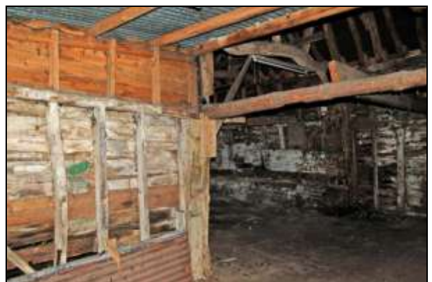
Plate 24: Pole at barn/extension juncture
