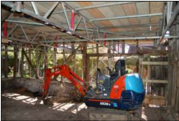
Plate 9: East wall during building works
