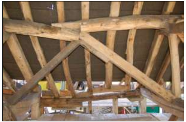
Plate 20: Edge halved scarf joints and purlin props
