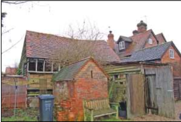
Plate 1: Barn and neighbouring privy from the east
