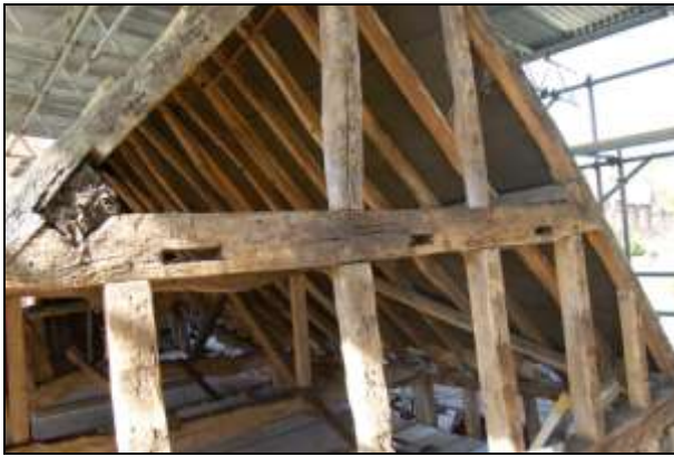
Plate 13: Mortices in north wall
