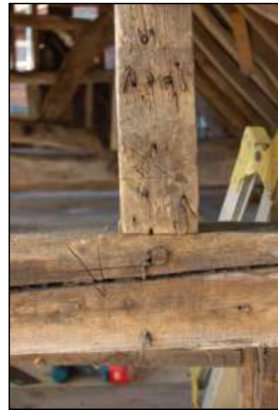
Plate 14: Carpenters assembly mark on north wall
