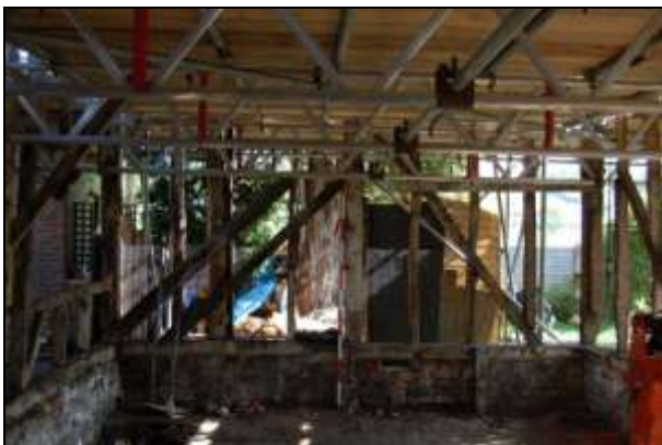
Plate 11: North wall during building works
