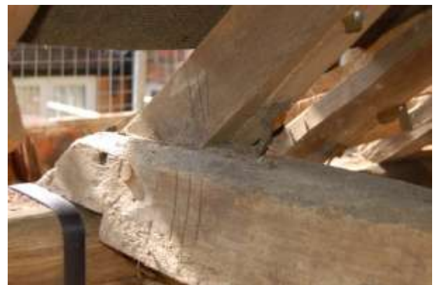
Plate 18: Carpenters assembly marks on Truss 1
