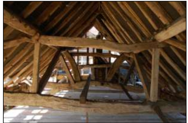
Plate 16: Trusses 1 and 2 from the scaffold
