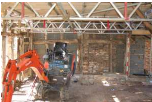
Plate 5: South wall during building works
