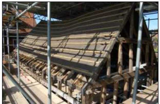
Plate 12: North wall and roof
