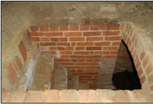
Plate 13: Detail of brickwork in the Smith burial vault
