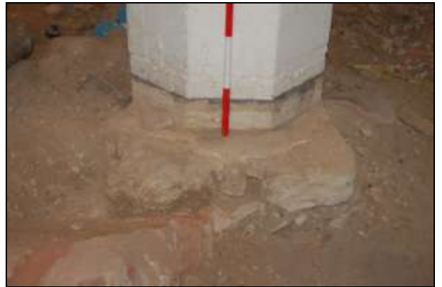
Plate 16: South aisle vault and truncated arcade column to the north
