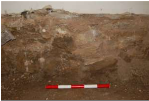
Plate 25: South chapel south wall fabric
