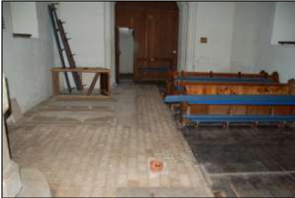
Plate 1: Brick, timber & cement flooring in the nave
