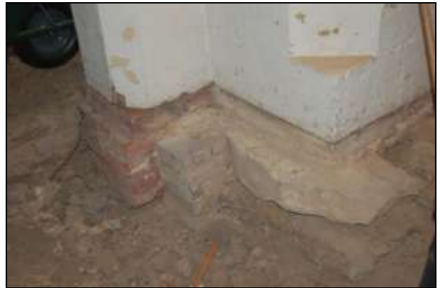
Plate 28: Brickwork supporting south side of chancel arch
