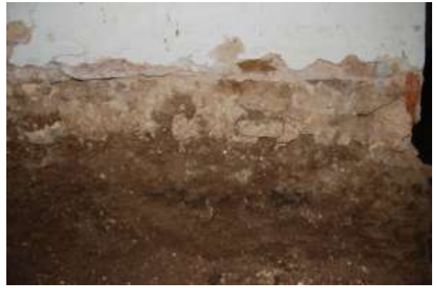
Plate 26: South chancel wall fabric
