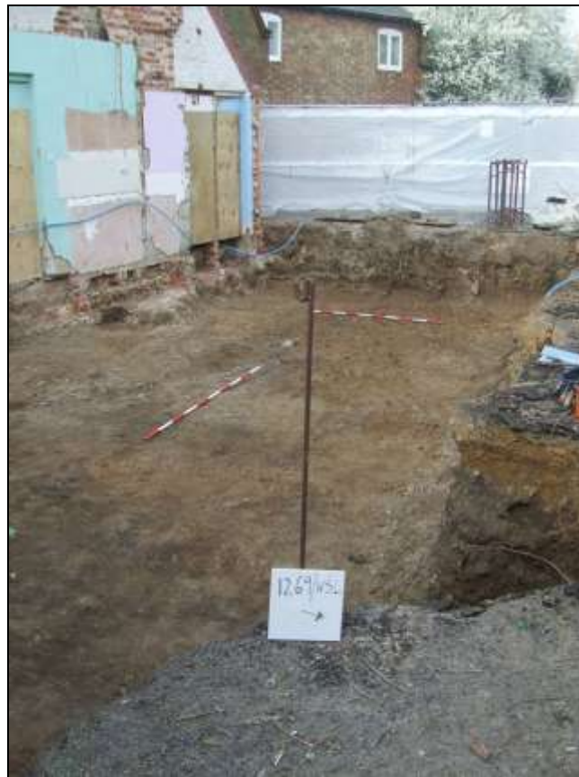
Plate 1: General site shot (scale 2×2m)
